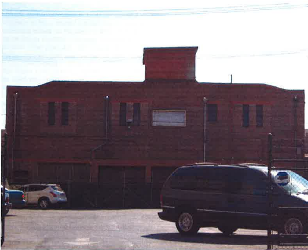
Rear (northeast) façade, looking southwest.
