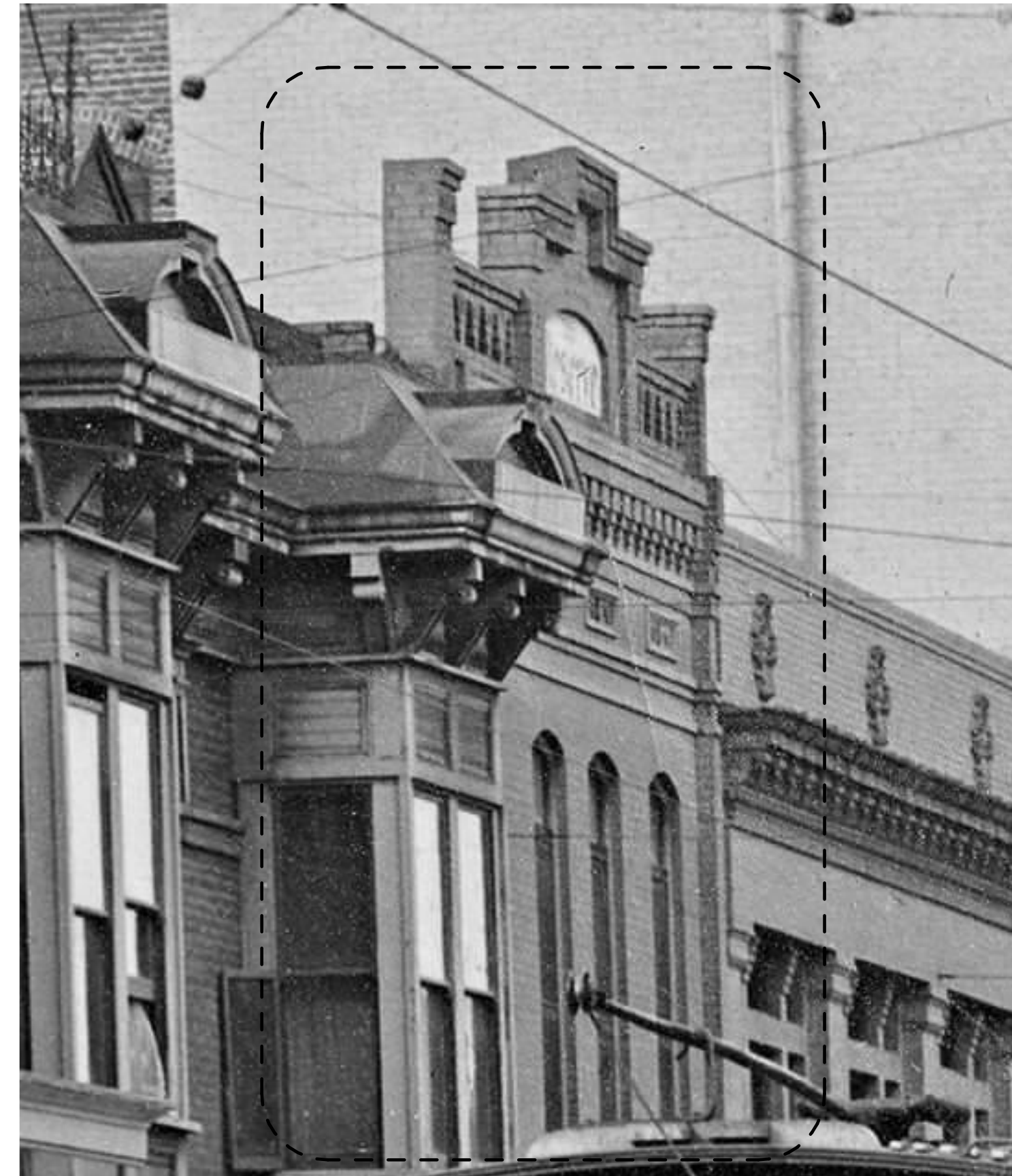
3 HISTORIC PHOTO OF SECOND FLOOR AND PARAPET FROM SOUTH
