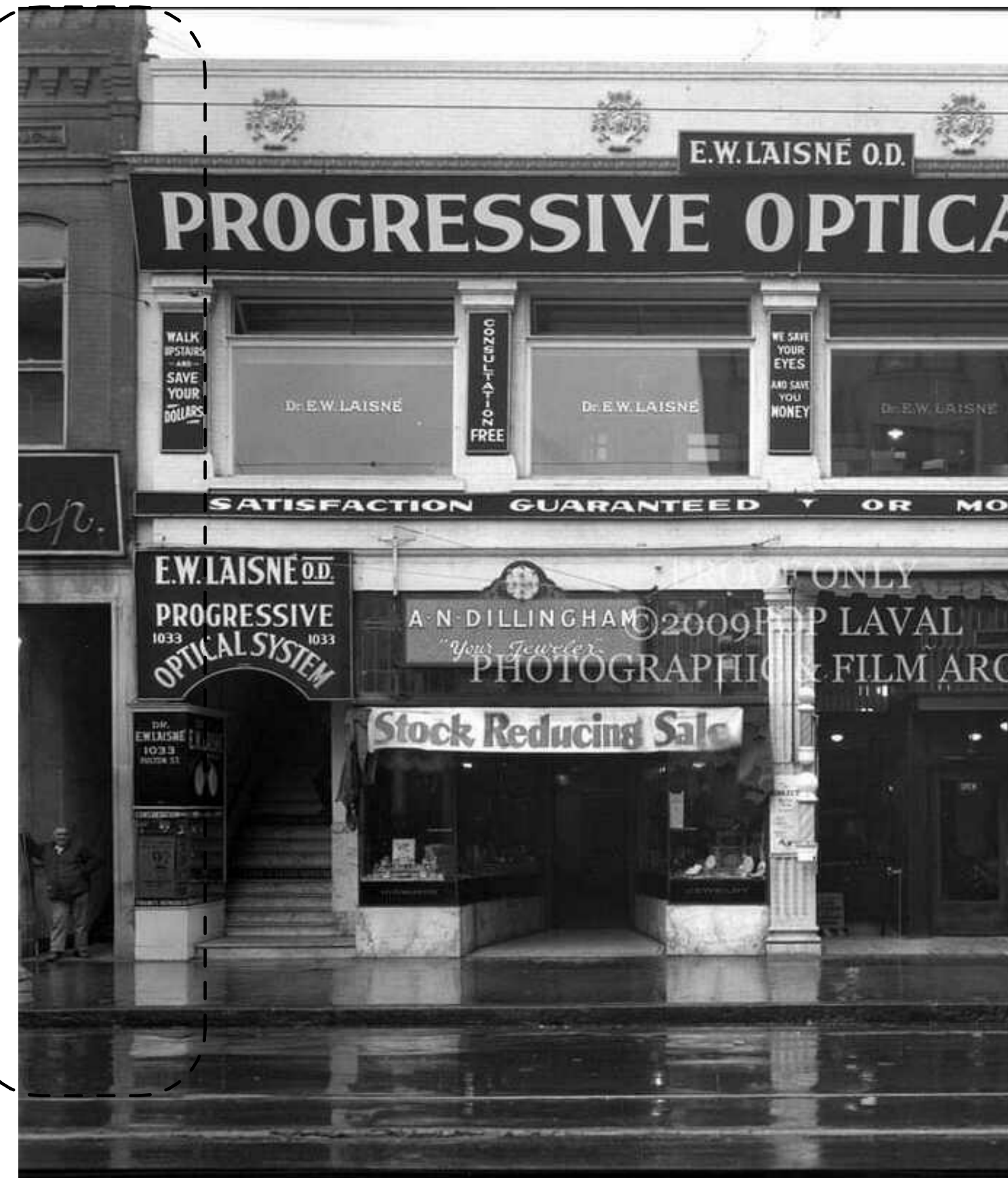
4 HISTORIC PHOTO OF FACADE NORTH EDGE
