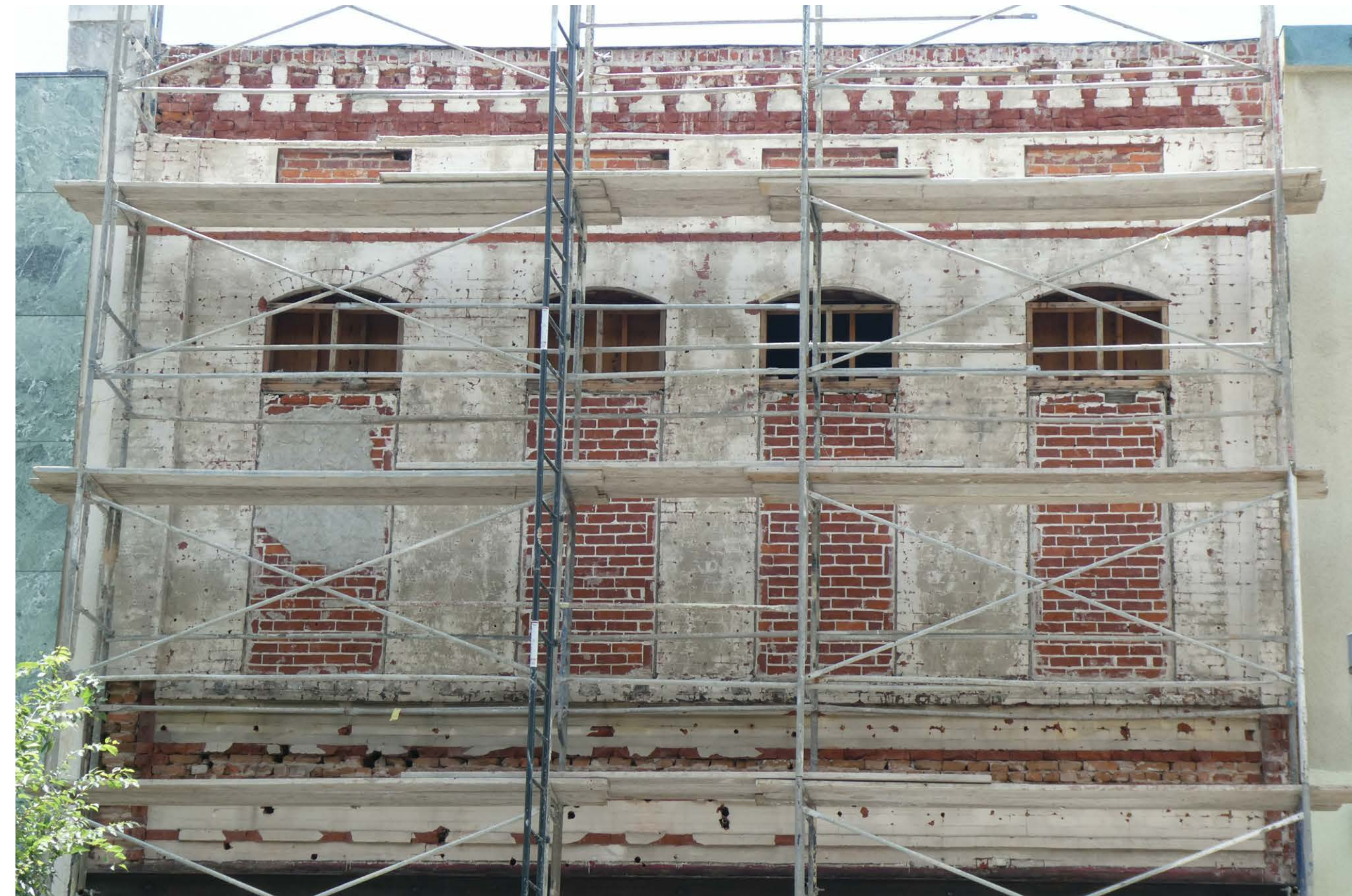
2 EXISTING CONDITION AT EAST FACADE MASONRY
