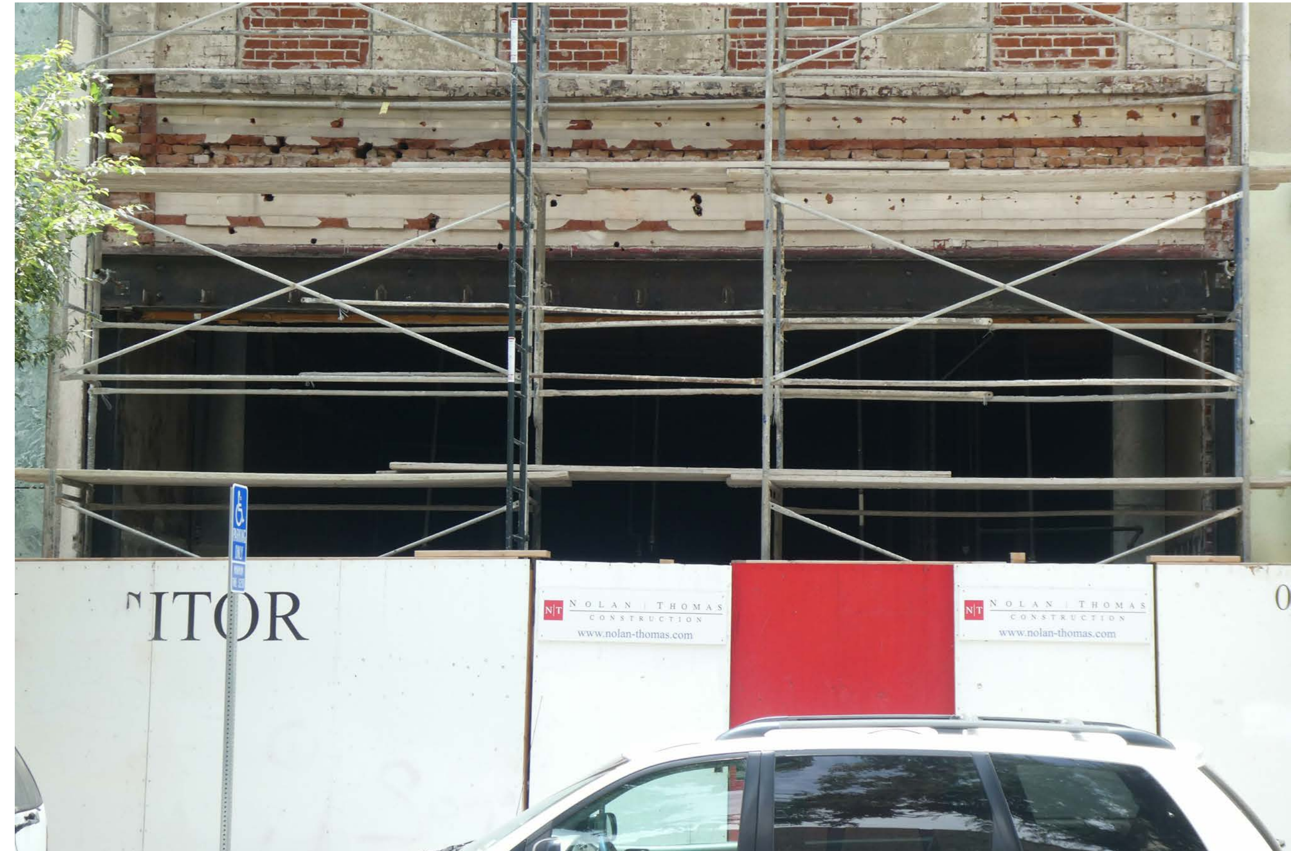
1 EXISTING CONDITION AT EAST FACADE STOREFRONT
