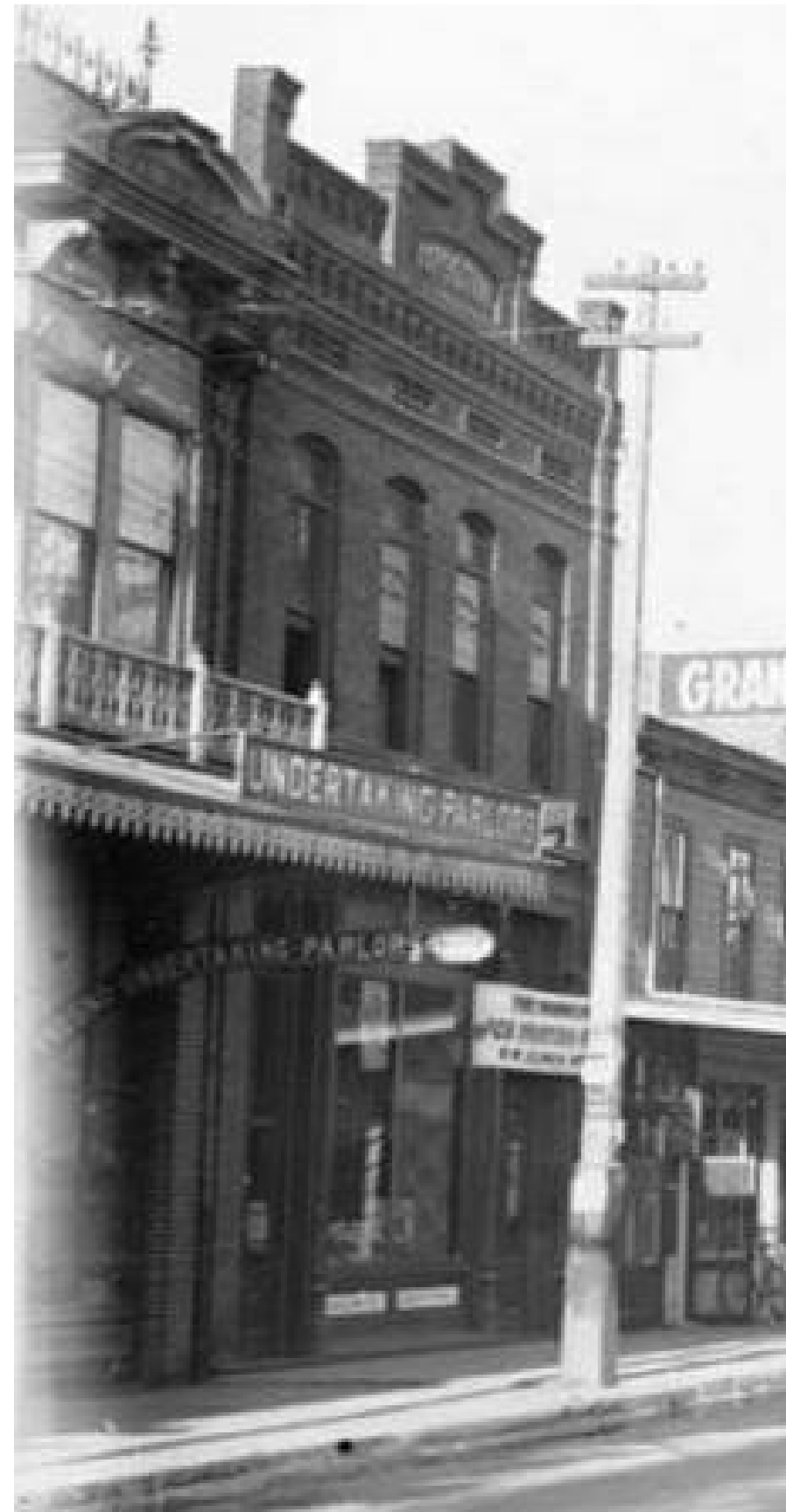
5 HIST. PHOTO OF FACADE FROM SOUTH
