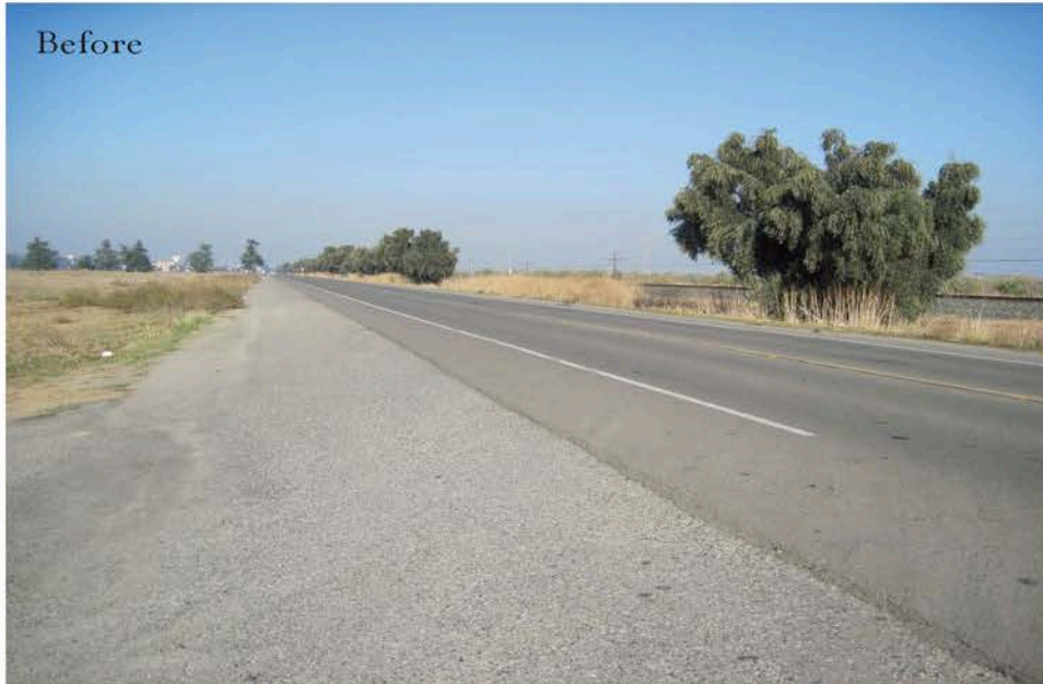
Looking north along Golden State Avenue at the location for the proposed Veterans Boulevard Interchange
