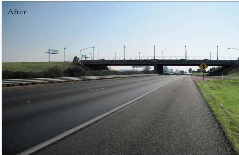
Looking south along State Route 99 at Veterans Boulevard Interchange
