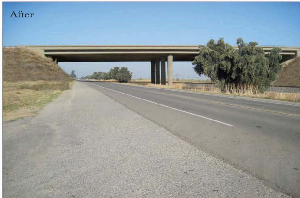
Looking north along Golden State Avenue at Veterans Boulevard Interchange
