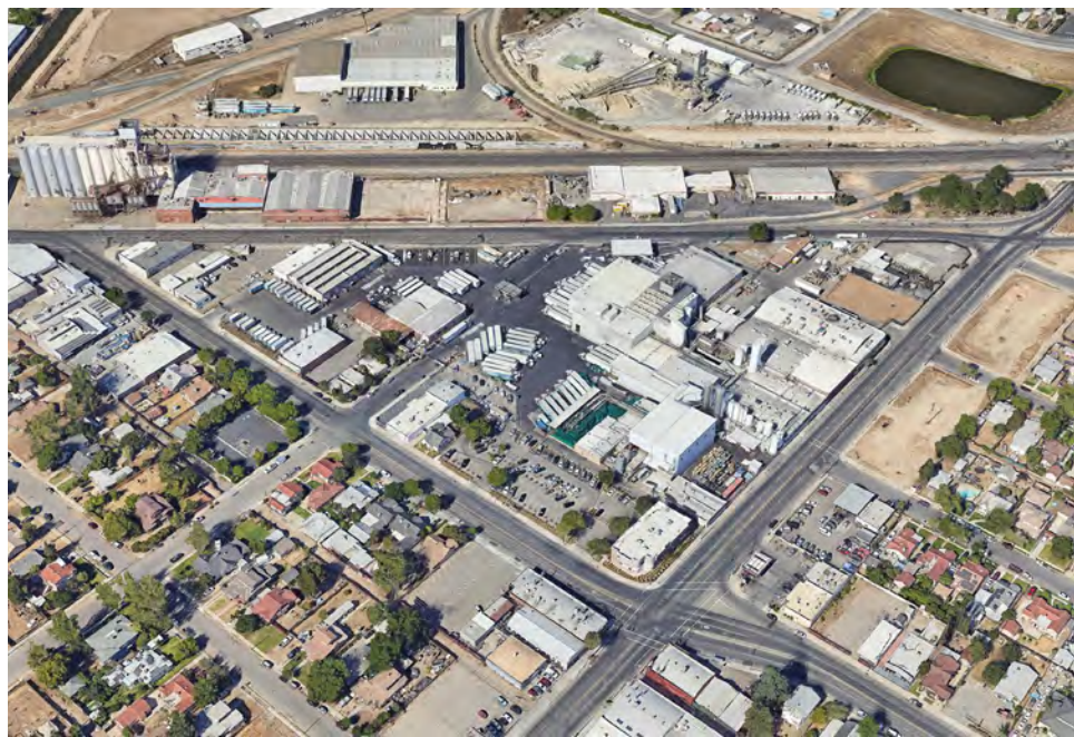
Aerial view of industrial cluster in southwest corner of plan area
