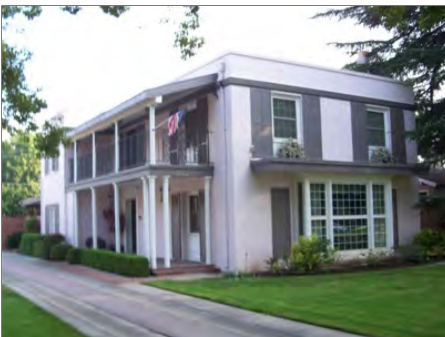
A house is rehabilitated with materials and finishes that are consistent with its original design.
