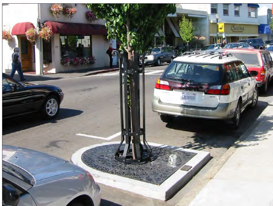
An in-street bulb-out brings the street tree closer to the automobile traffic, narrowing the perceived width of the street while allowing an uninterrupted pedestrian path along the sidewalk.
