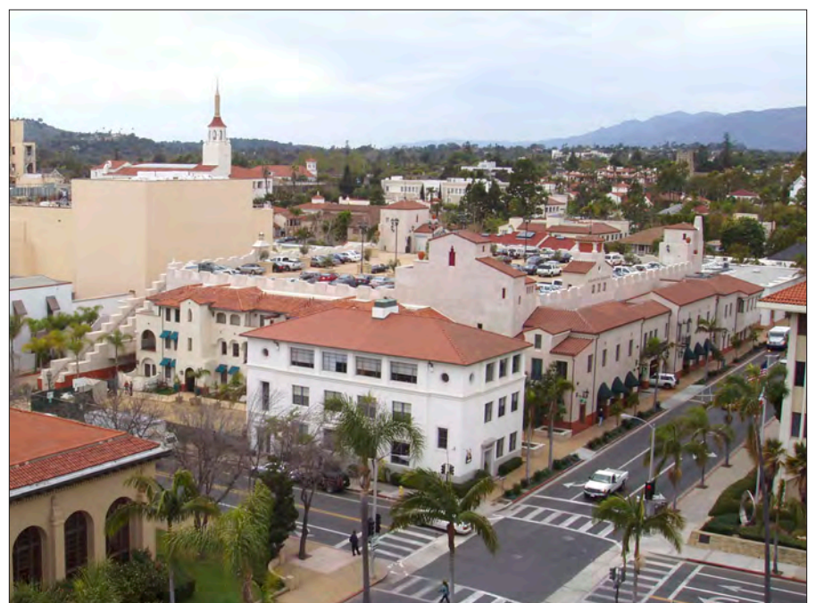
Parking is placed in a garage that is lined with street-facing retail and/or office uses to create an active streetscape that would otherwise be dominated by automobile parking.
