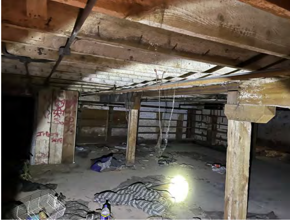
PHOTO # 19 COMMENTS : South basement floor framing. Unconventional floor beam supports.
