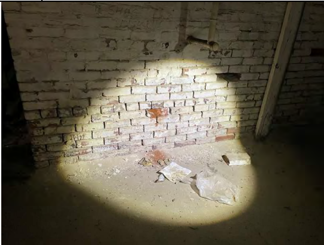
PHOTO # 18 COMMENTS : Basement wall brick and mortar deterioration. The brick on the floor was easily removed by hand.
