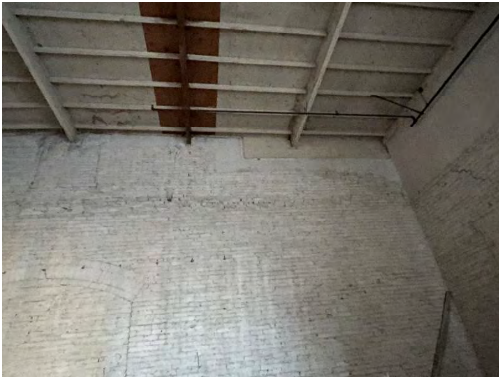
PHOTO # 4 COMMENTS : View of roof purlins supported at the north end wall and glu-lam outrigger beam. Note the newer unpainted roof plywood and purlin.
