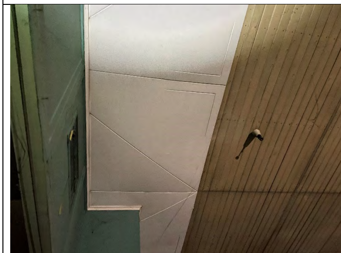
Pressed Wood Panel Ceiling
