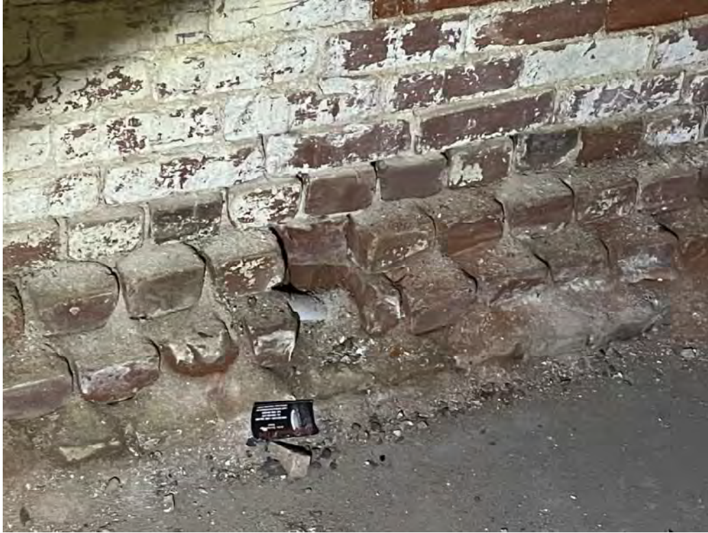
PHOTO # 15 COMMENTS : View of the bottom of a portion of the basement wall. Extreme brick and mortar deterioration.
