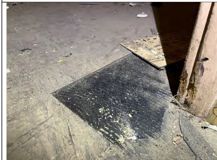
Black and Yellow Mastic Under Floor Tile
