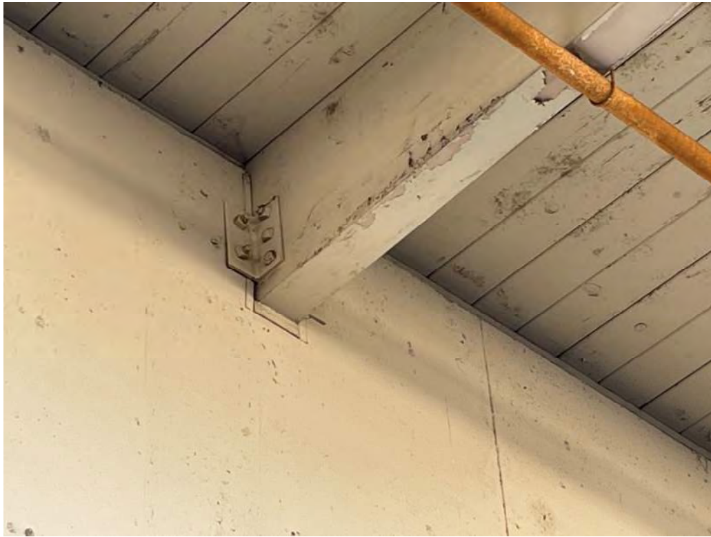
PHOTO # 11 COMMENTS : Glu-lam girder extending through pocket in exterior wall. Note the clip angle bolted to the wall and beam (each side). This is the only method of connection of the exterior walls to the roof structure.
