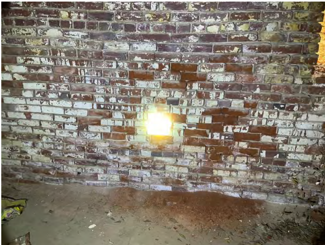
PHOTO # 16 COMMENTS : A typical basement wall surface with extreme brick and mortar deterioration. Note the 'Red Dust' piled at the bottom of the wall. Evidence of a very long term condition beyond repair.
