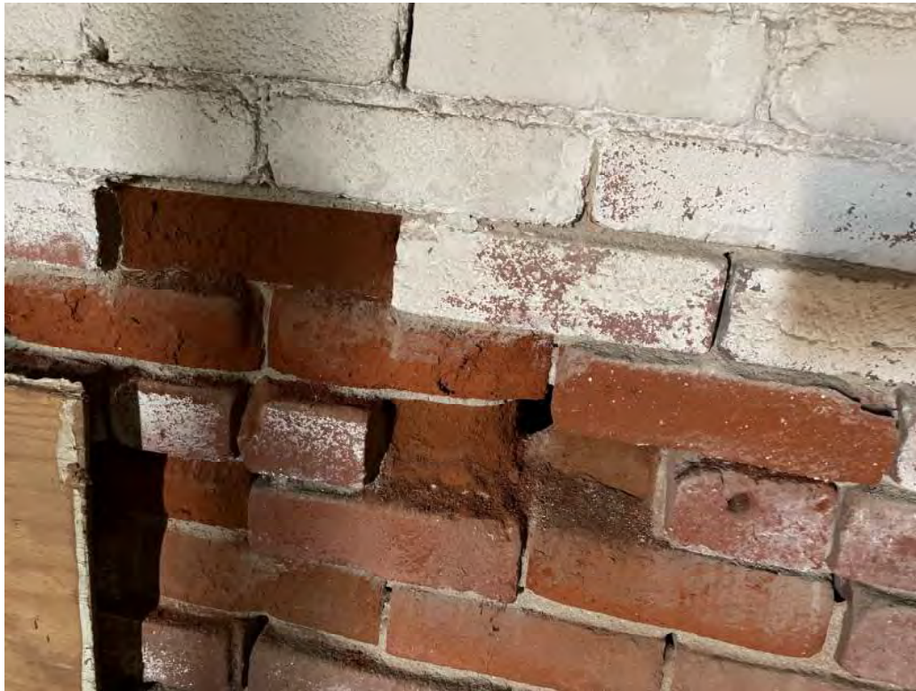
PHOTO # 7 COMMENTS : Brick exfoliation at interior surface of the west wall. Note the extreme degree of deterioration of both brick and mortar.
