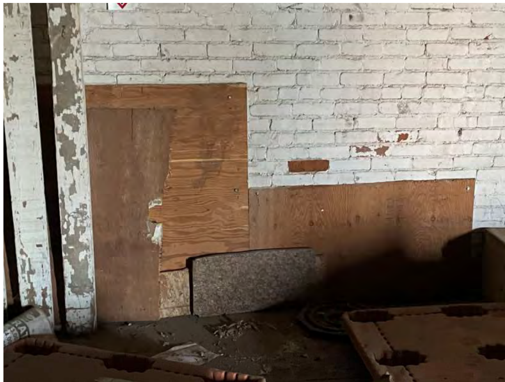
PHOTO # 8 COMMENTS : Interior of west wall with plywood to cover over extreme deteriorations of the brick and mortar.
