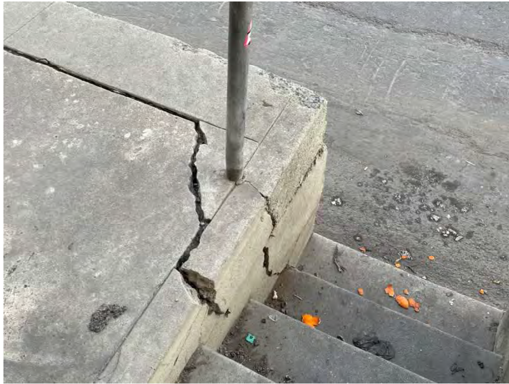
PHOTO # 31 COMMENTS : Failure of the concrete slab breaking away from the loading dock at the H St. wall.
