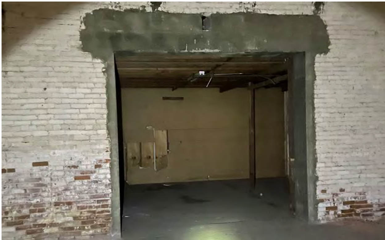
PHOTO # 12 COMMENTS : Interior opening between areas of the building. Note the grout at the header indicating a repair or replacement of the original header system.
