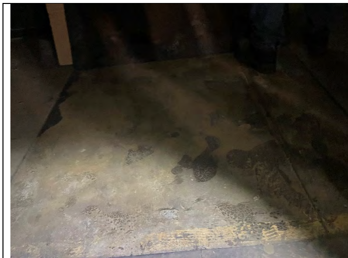
Black and Yellow Mastic Under Floor Tile
