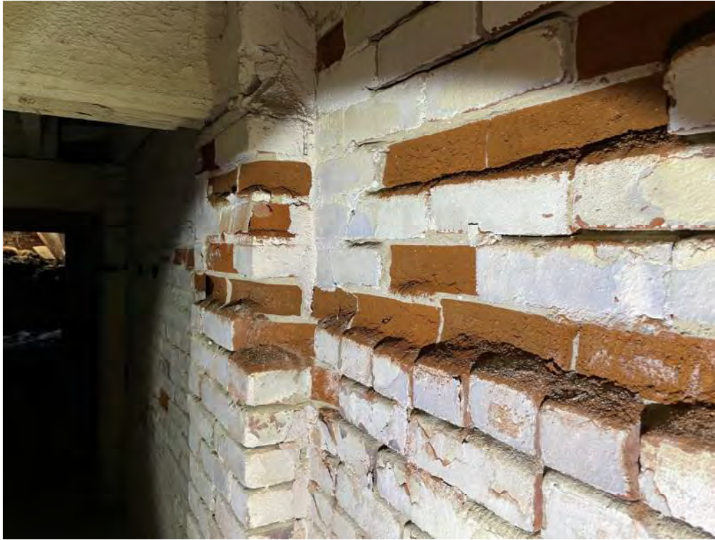
PHOTO # 17 COMMENTS : Basement wall deterioration in pilaster supporting a main floor beam.
