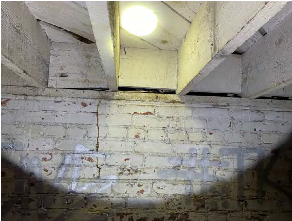
PHOTO # 20 COMMENTS : View of floor joists setting on basement wall wood plate. Blockings between joists do not have connections to the wood plate. Not shear resistance exists between the floor and the basement wall.
