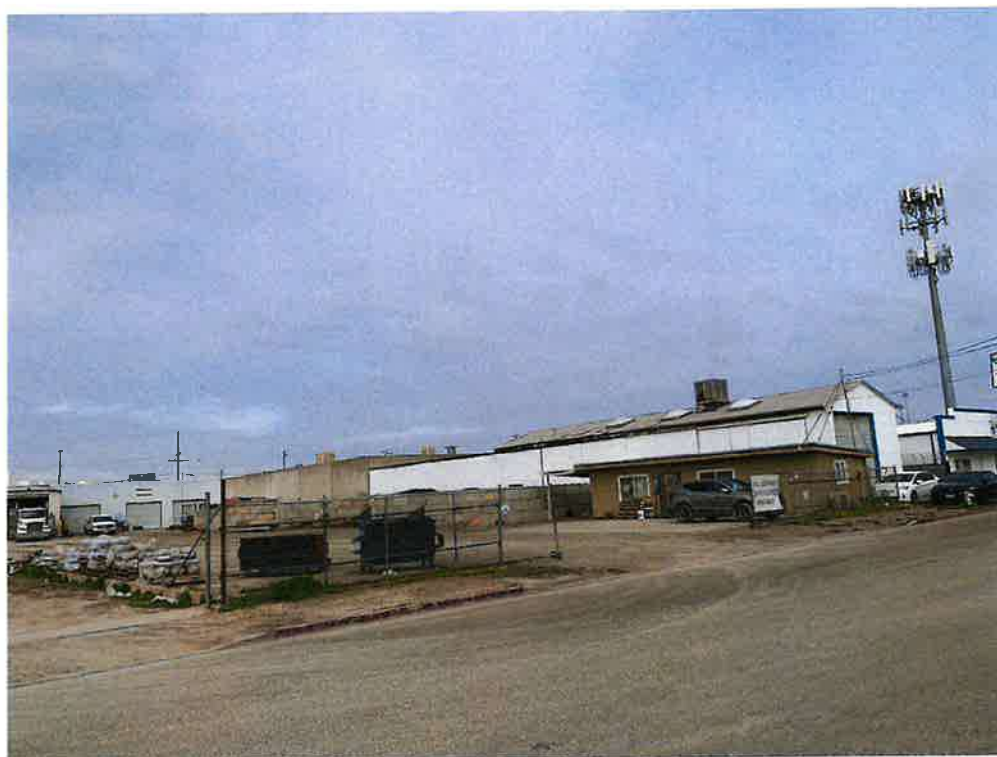
ENTRANCE FROM N. EFFIE
