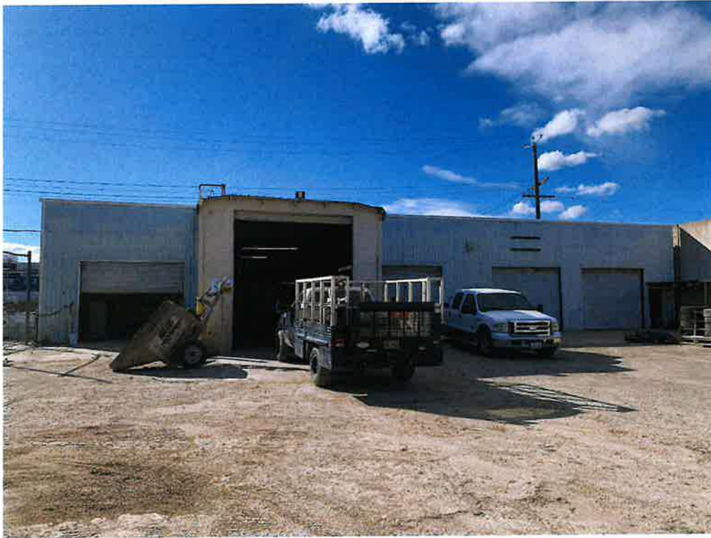
MAINTENANCE SHOP EXTERIOR
