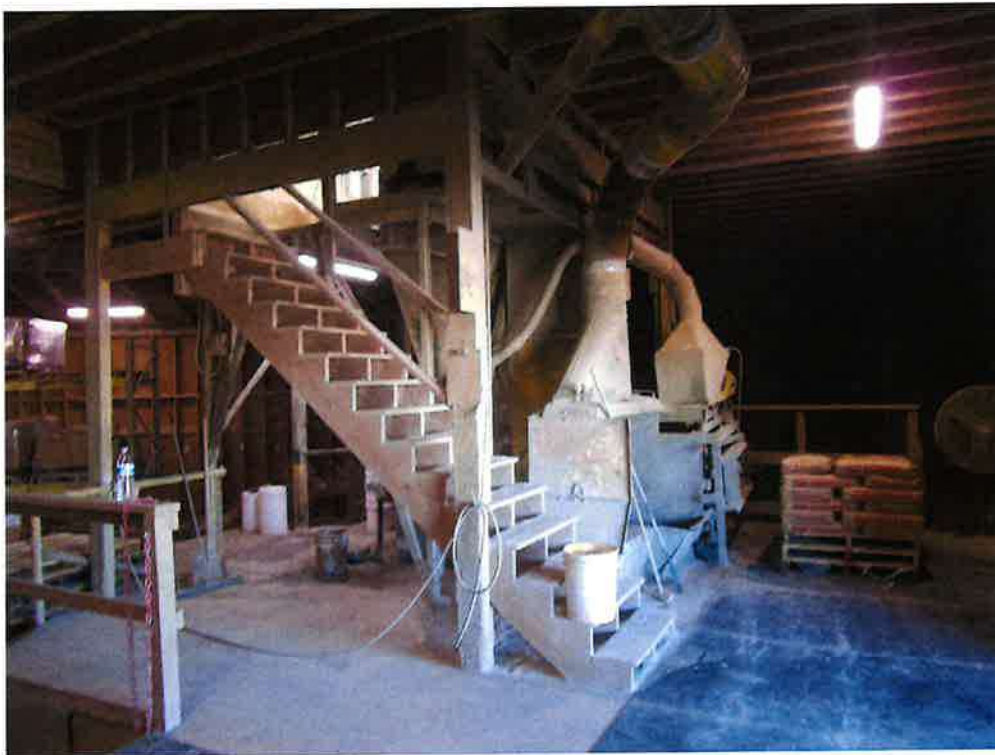
STUCCO MANUFACTURING PLATFORM & EQUIPMENT
