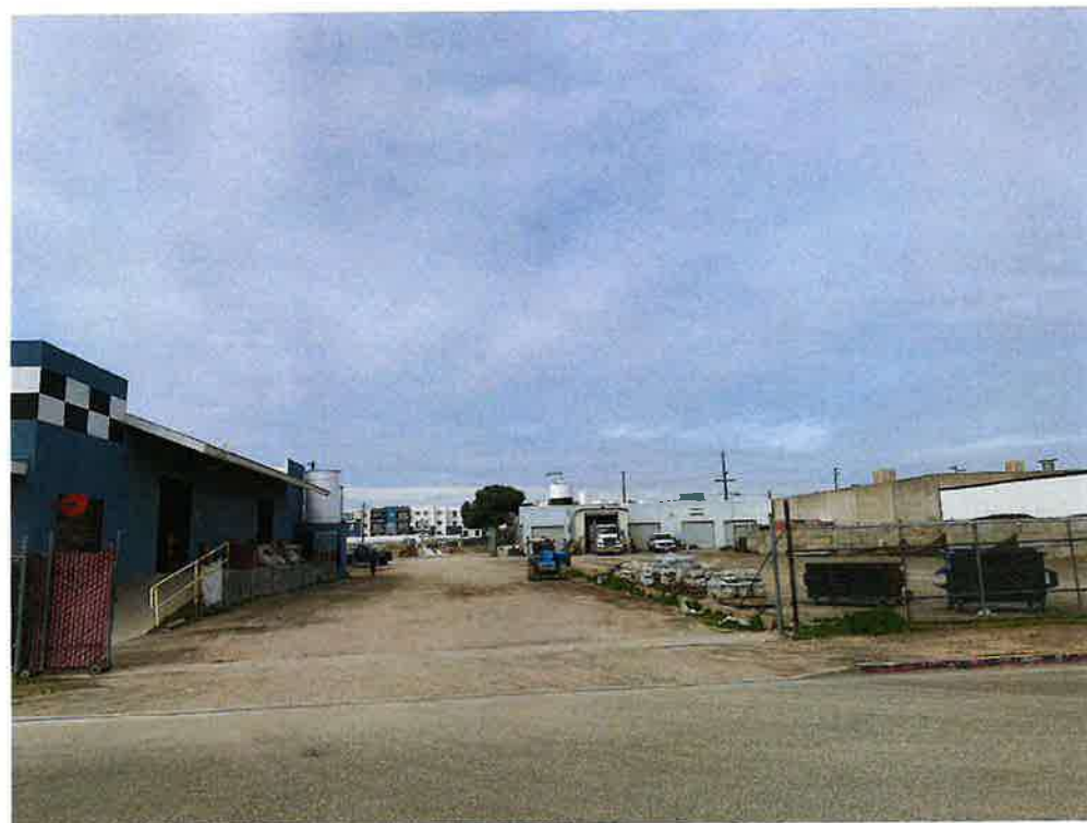
OVERALL SUBJECT PROPERTY
