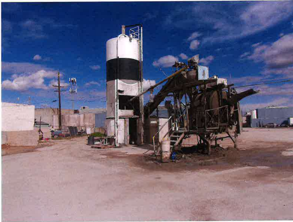
CONCRETE BATCH PLANT
