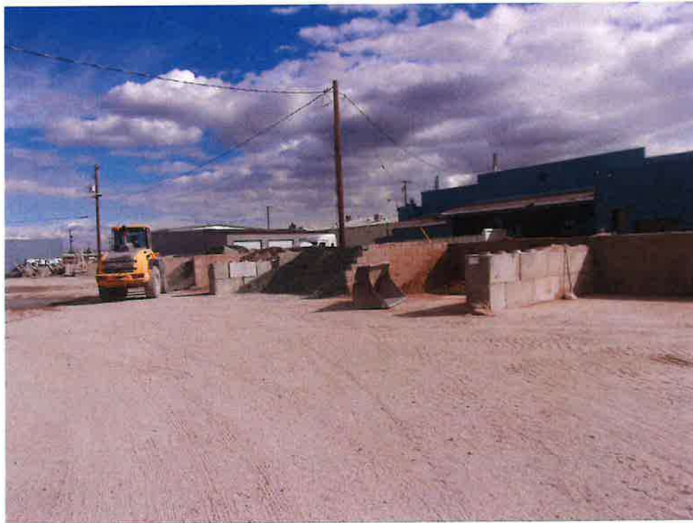
MATERIAL SCALE HOPPER & CONVEYOR
