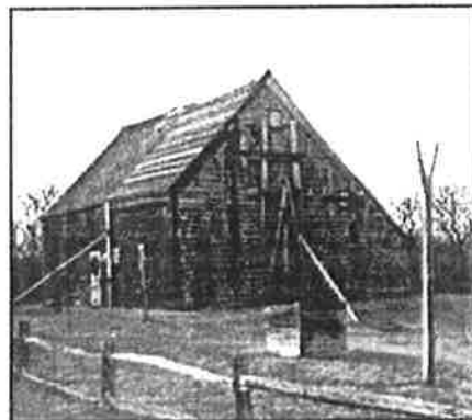
Buildings seriously damaged by storms or deterioration may need to be braced before architectural evaluations can be made. Photo: John Milner Architects. Photo: NPS files
