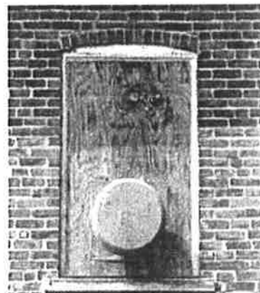
This exhaust fan has tamper-proof housing. Photo: Michael Mills, Ford Farewell Mills Gatsch, Architects.
