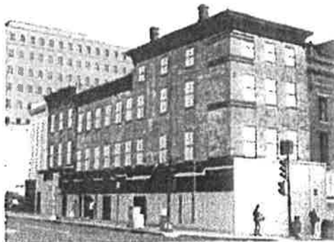
Urban buildings often need additional protection from unwanted entry and graffiti. This commercial building uses painted plywood panels to cover its glass storefronts. The upper windows on the street sides have been painted to resemble 19th century sash. Photo: NPS files.
