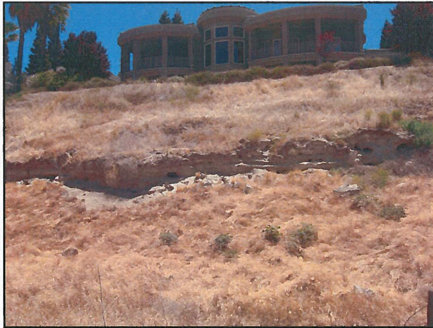
Photo No. 4. Eroded Section of Perrin Ditch in the Project Area
