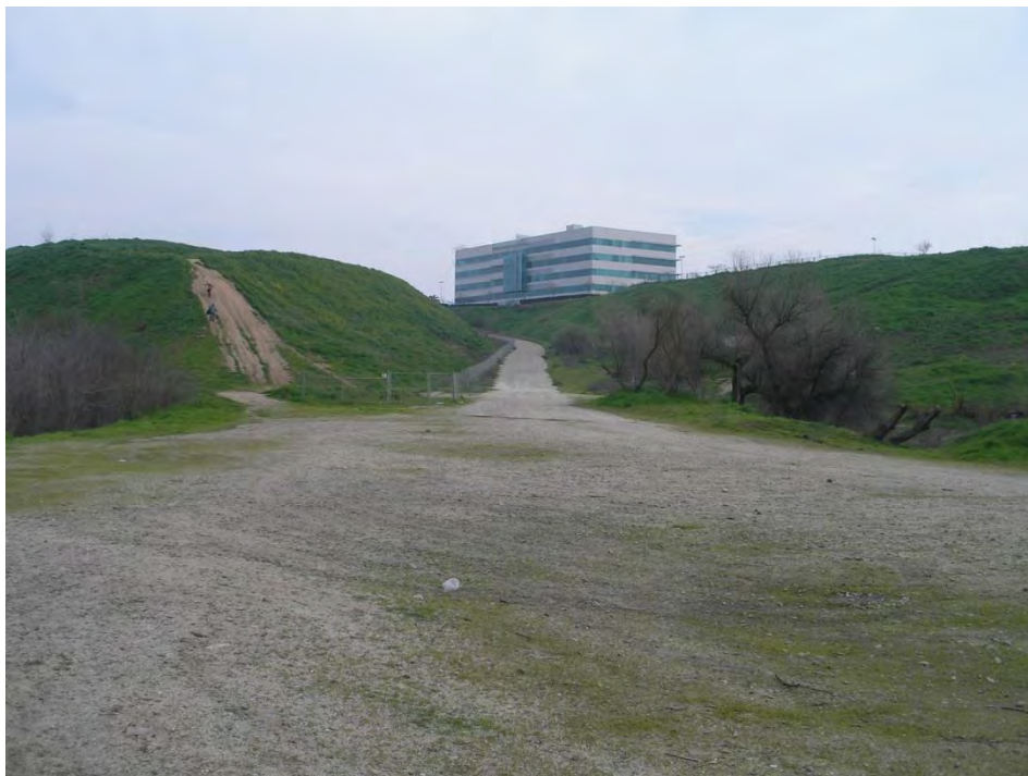
Photograph 2. View of paved Gravel Haul Road facing the Park Place Shopping Center located on bluff.
