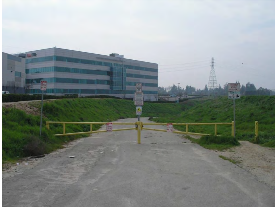
Photograph 5. Locked entrance to the area. View is looking toward the west.
