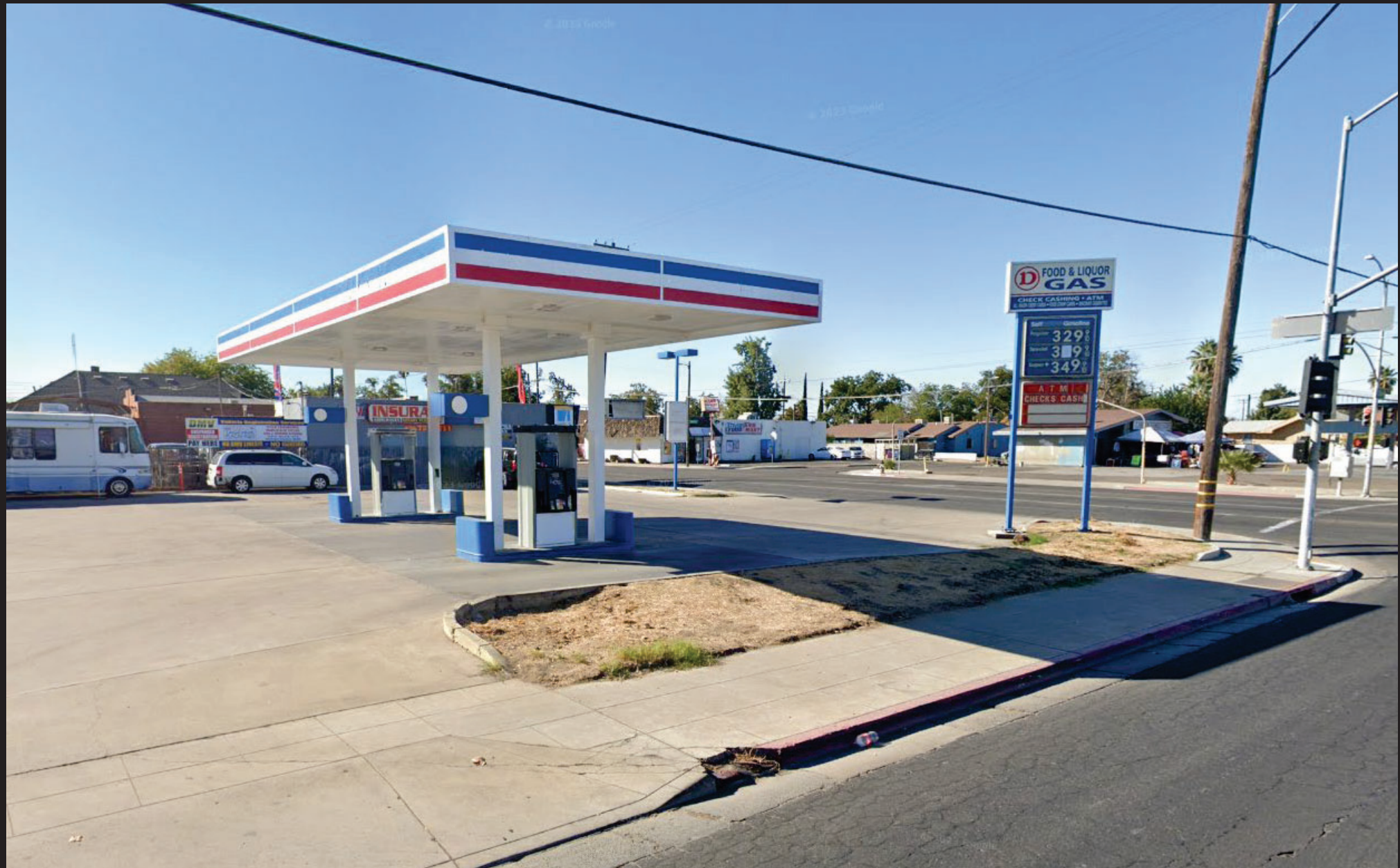
Canopy & Gas Pumps – 2520 E. Olive Ave.
