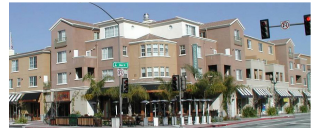
Mixed-Use Building. Within a Mediterranean style vocabulary, residential uses are located on the upper two floors, while the retail is at the street-level.
