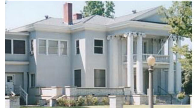
Neo-Classical Example. Neo-classical facades commonly use columns, triangular pediments (the ends of gabled roofs), and symmetrical arrangements.
