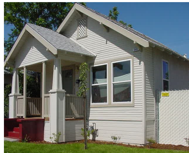
Renovated Façade on Palm Avenue Bungalow.
