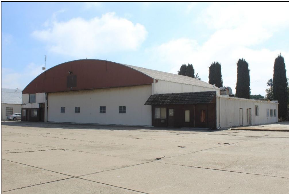
Figure 4. North and west façades of the hangar, facing southeast (Stantec, 2025).
