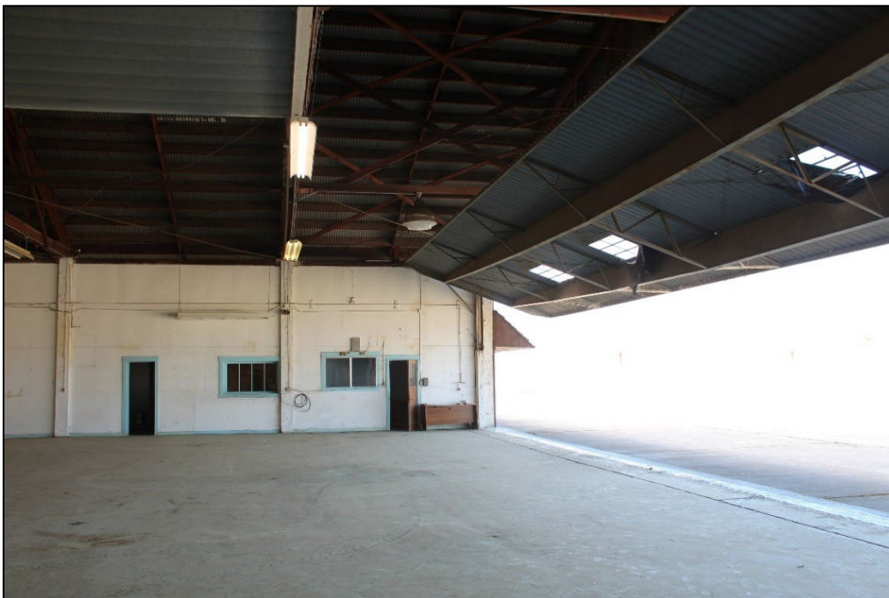
Figure 12. Interior of the hangar with hangar door open, facing west (Stantec, 2025).
