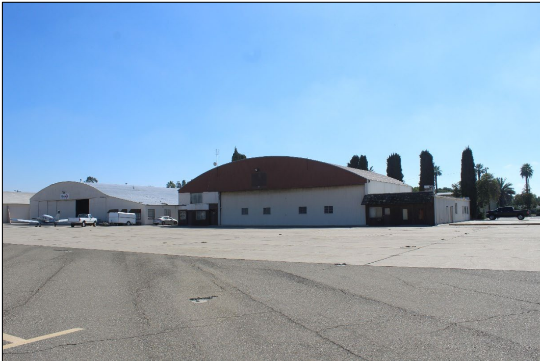
Figure 2. Hangar at 716 W. Kearney Boulevard within the Fresno Chandler Executive Airport, facing southeast (Stantec, 2025).
