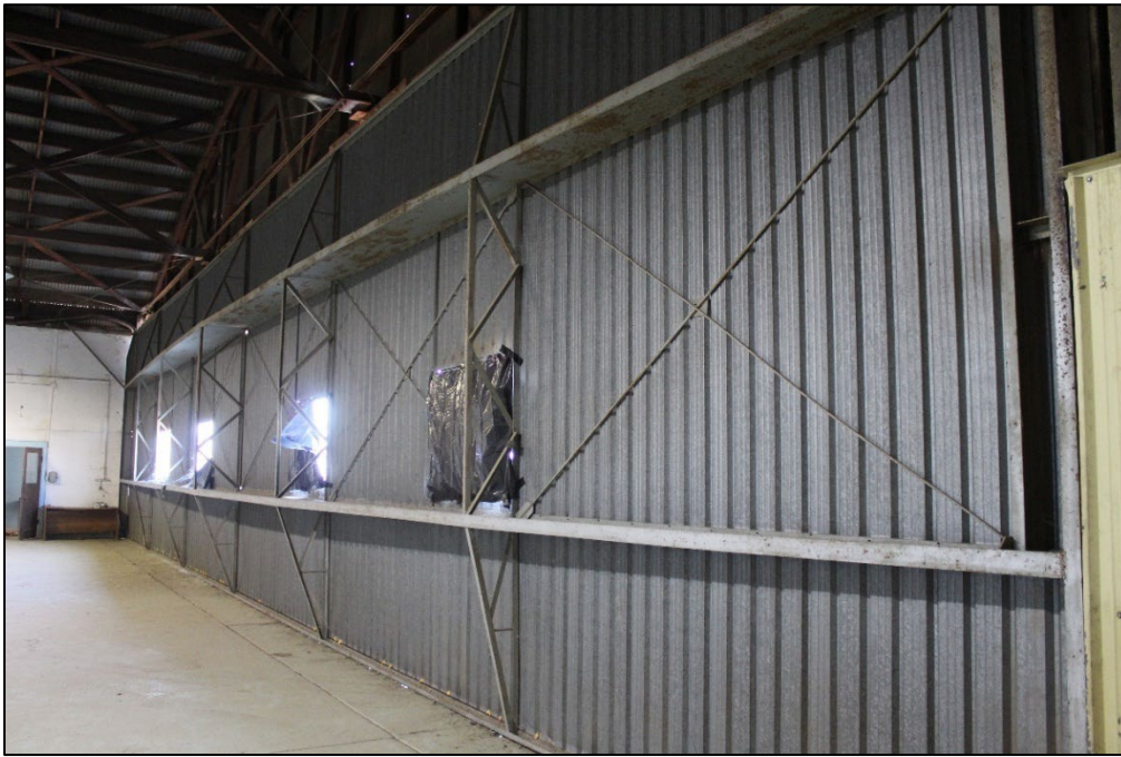
Figure 15. Interior of hangar with hangar door closed, facing west (Stantec, 2025).
