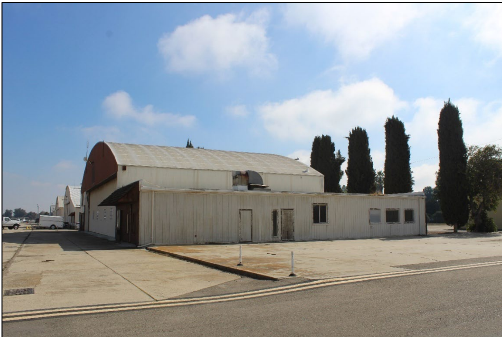
Figure 6. West façade of the hangar, facing east (Stantec, 2025).
