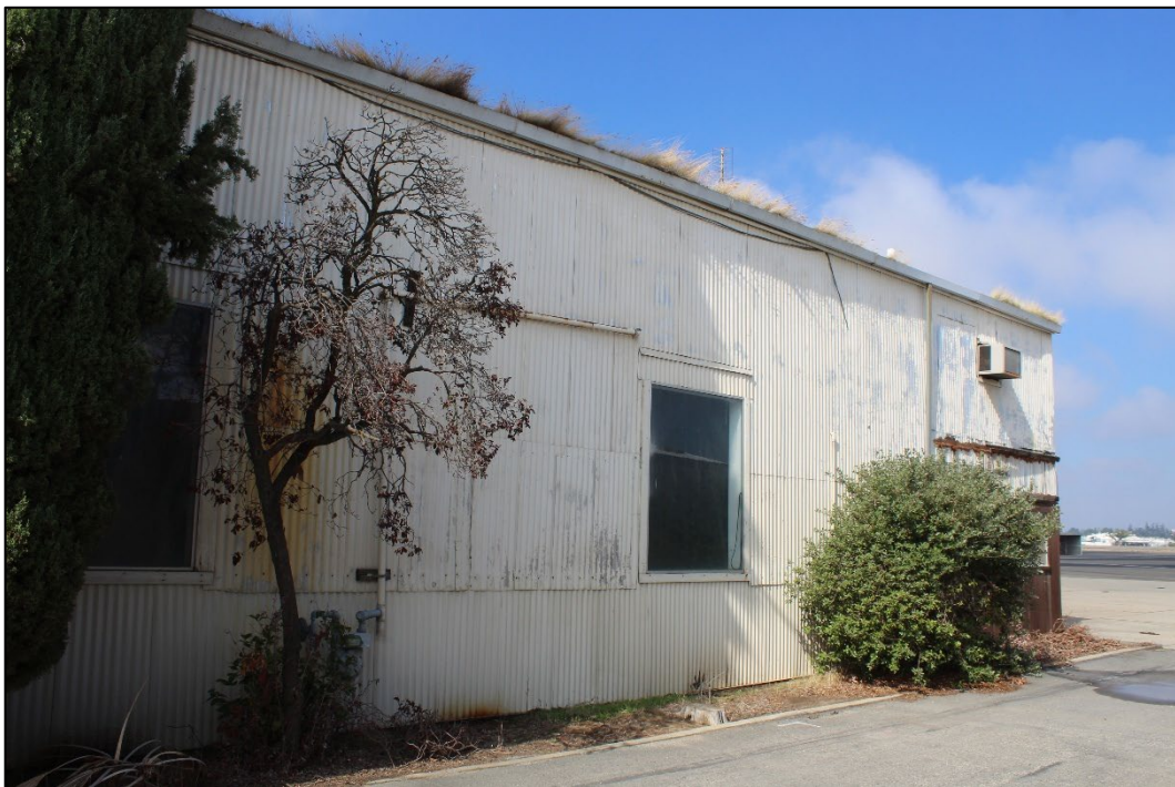
Figure 13. East façade of the hangar, facing northwest (Stantec, 2025).
