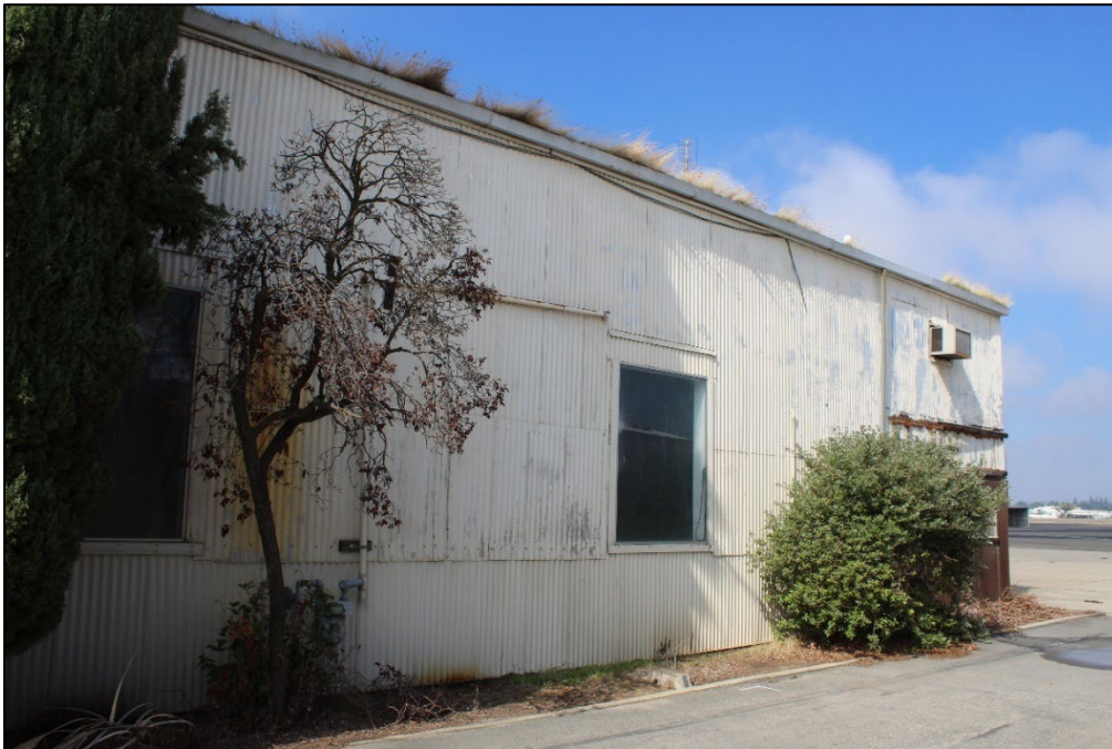
Figure 11. East façade of the hangar, facing northwest (Stantec, 2025).
