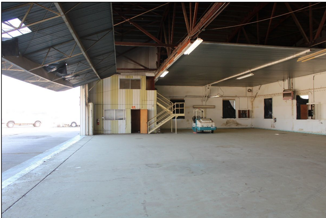
Figure 15. Interior of the hangar with hangar door open, facing east (Stantec, 2025).
