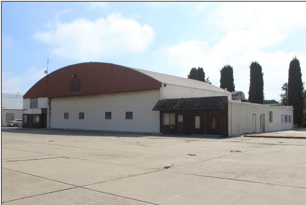
Figure 6. North and west façades of the hangar, facing southeast (Stantec, 2025).
