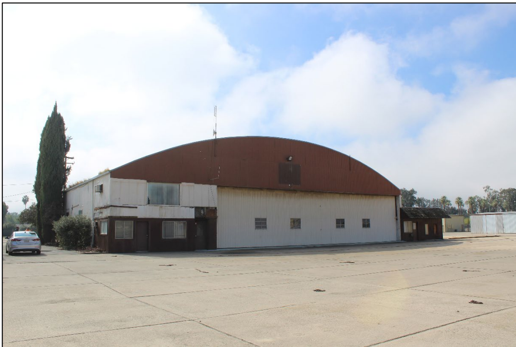
Figure 3. North façade of the hangar, facing southwest (Stantec, 2025).
