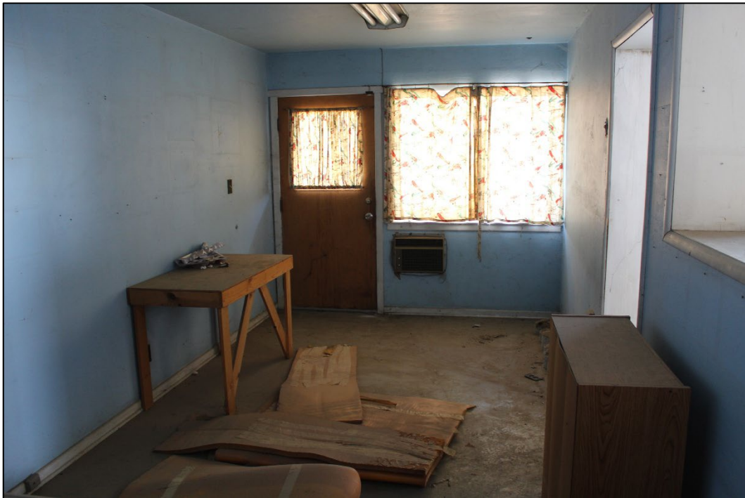
Figure 22. Interior of the addition, facing north (Stantec, 2025).
