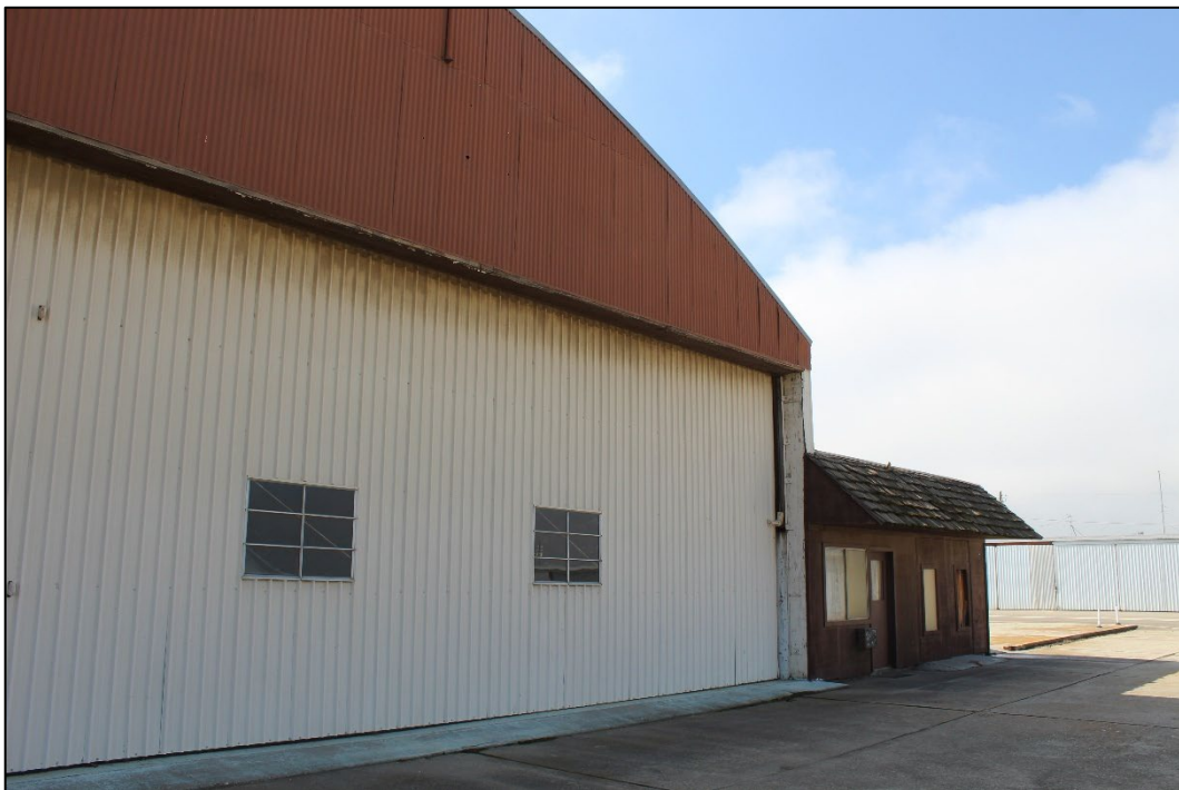
Figure 5. West end of the north façade of the hangar, facing southwest (Stantec, 2025).
