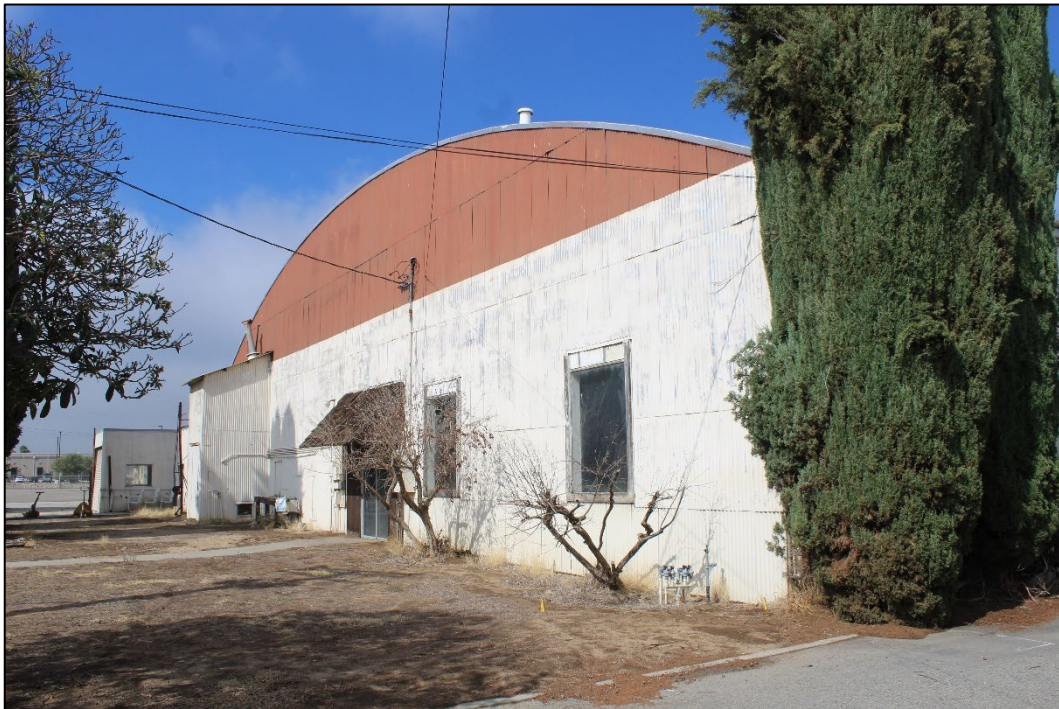
Figure 12. South façade of the hangar, facing northwest (Stantec, 2025).
