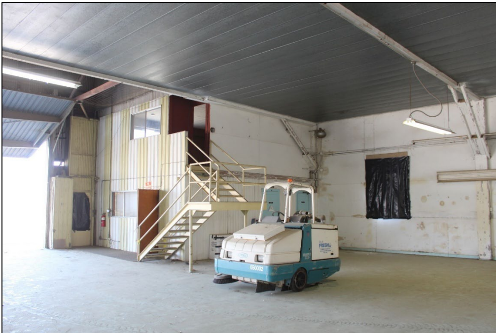
Figure 16. View of the integrated office and apartment from inside of the hangar, facing northeast (Stantec, 2025).
