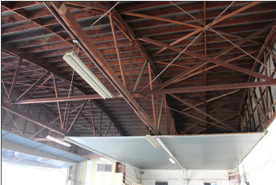
Figure 16. Wood truss frame roof inside the hangar (Stantec, 2025).
