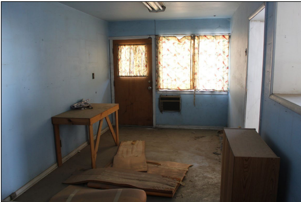
Figure 20. Interior of the addition, facing north (Stantec, 2025).
