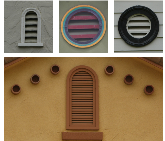
Attic Vents. Common attic vent types in the Tower District.
