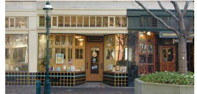
Recessed Storefront Entrance. Doors into retail spaces may be recessed within the façade, so doors don’t swing into sidewalks, and entry should be at same grade as the adjacent sidewalk.
