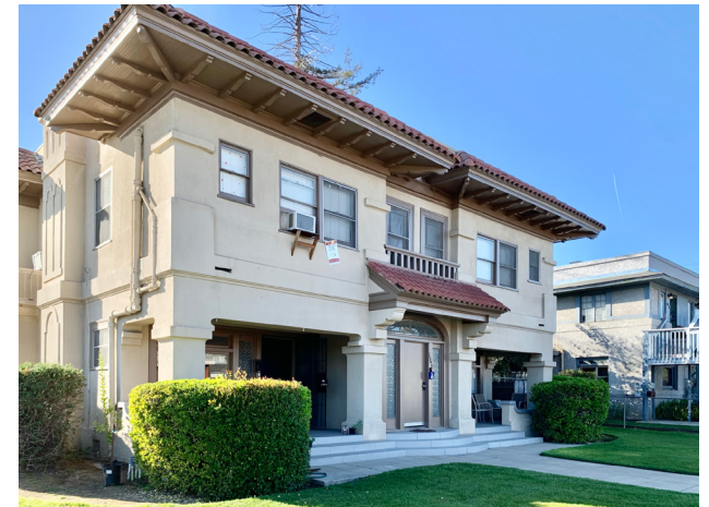
Small four unit apartment building at Wishon and McKinley.
