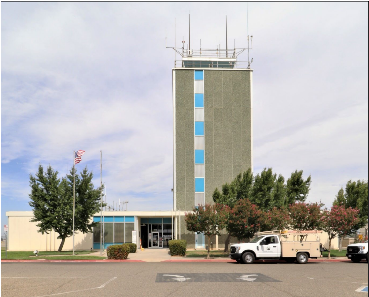
Photo 1: Southwest elevation, view northeast (9/11/23).
