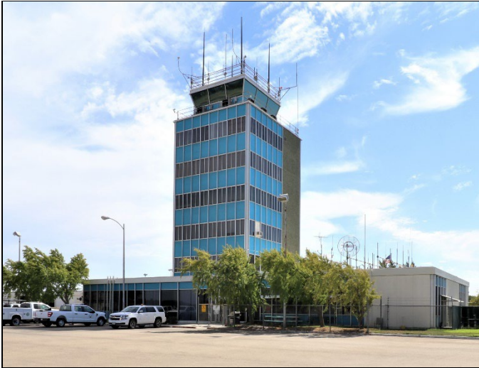
Northeast elevation, view south (9/11/23).
