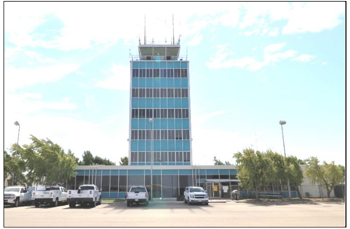
Northeast elevation, view southwest (9/11/23).
