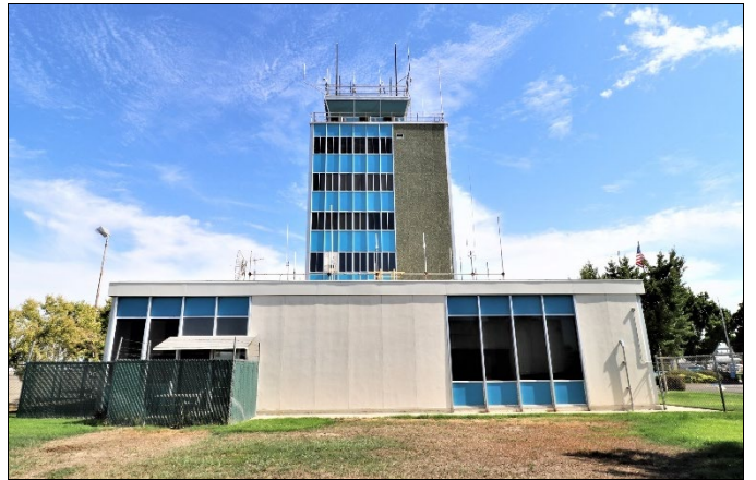
Northwest (side) elevation, view southeast (9/11/23).
