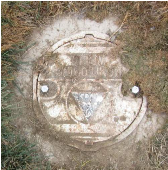
Photo 25: "C" Zone Monitoring Well
