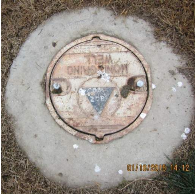
Photo 24: "B" Zone Monitoring Well
