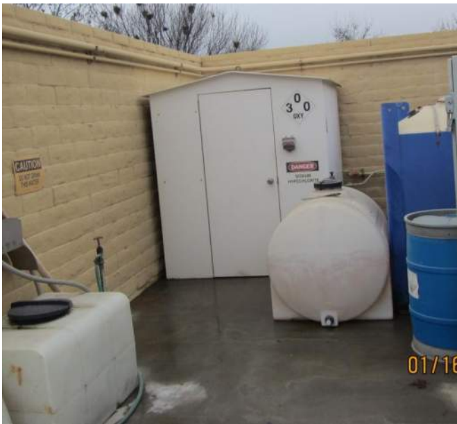
Photo 9: Hazardous Materials Storage Shed
