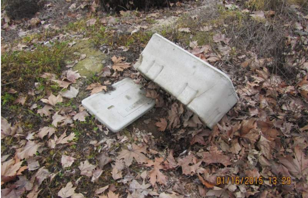
Photo 10: Evidence of Electrical Components Theft
