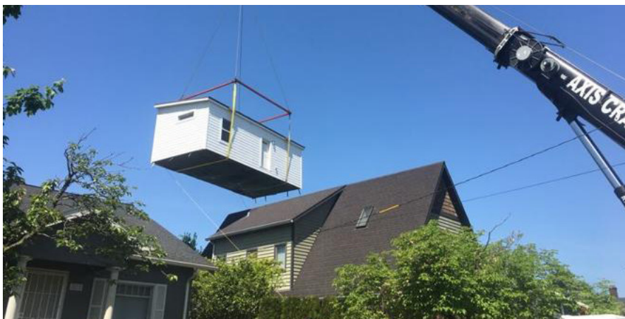
An example of a prefabricated ADU 1 being craned into a residents backyard.
