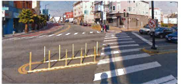
Fig 3.14: Example of soft-hit posts as median-refuges (source: Google Streetview)
