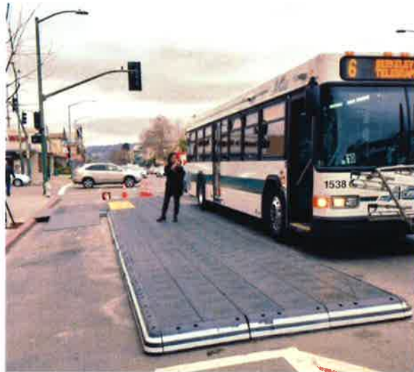
Figures 3.20: Temporary Boarding Island in Oakland, CA
