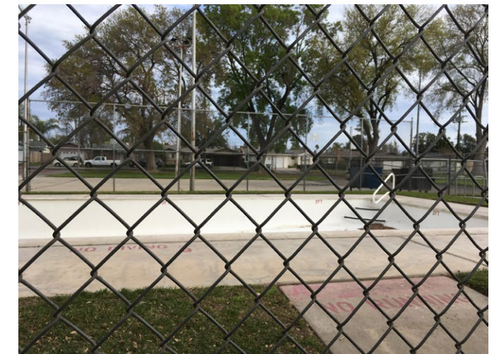
Rarely used pool in disrepair and not very functional for use
