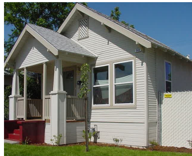
Renovated Façade on Palm Avenue Bungalow.
