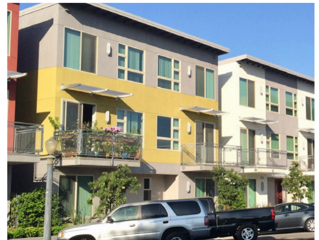
Street-Oriented Apartments. Contemporary multifamily development lines streets in a pedestrian-friendly way near the Tower District.
