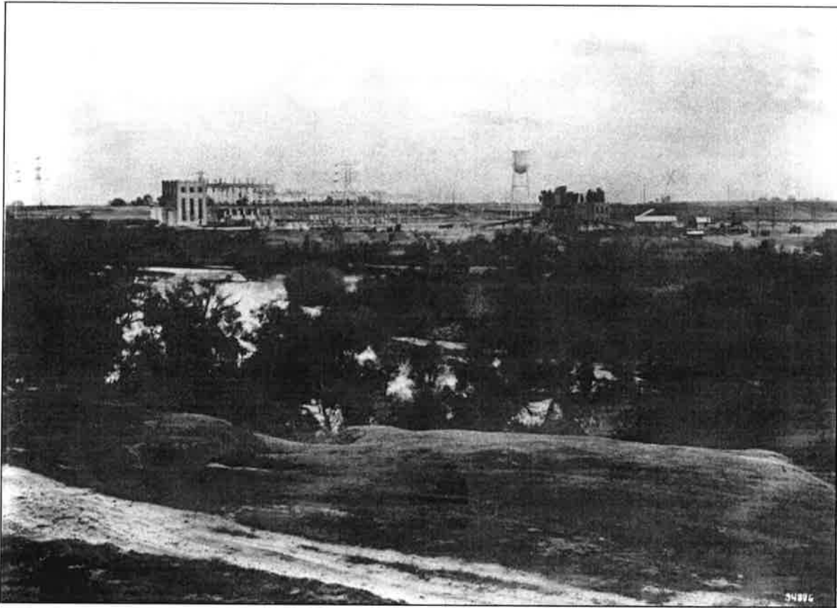
Figure 3-1 View from the north side of the San Joaquin River in Madera County documenting the completed Herndon Substation in 1931 (photo on file, General Maintenance Orders, PG&E Archives, Brisbane, California).
