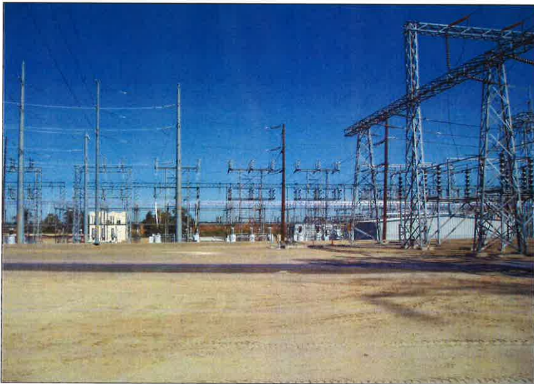
Figure 4-3 View from the same angle illustrating the changes at the substation in the last 77 years (Applied EarthWorks, August 2008).
