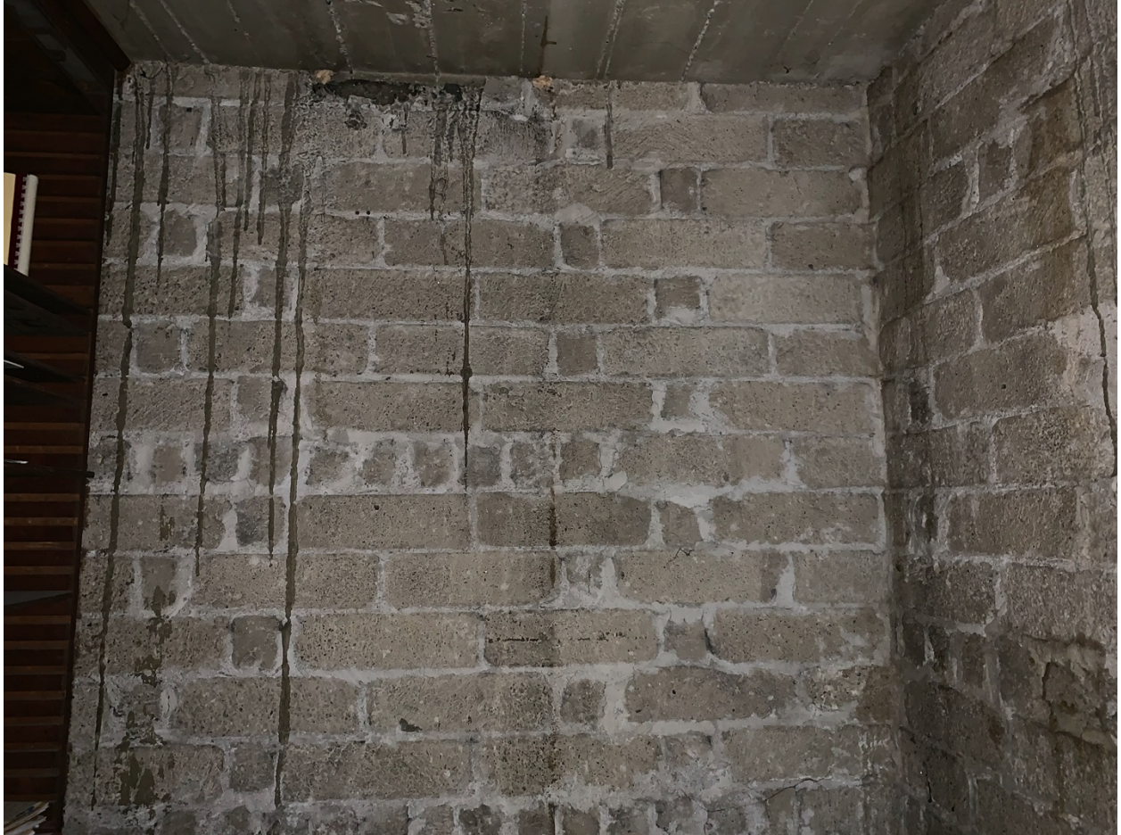
Existing interior photo of original brick
