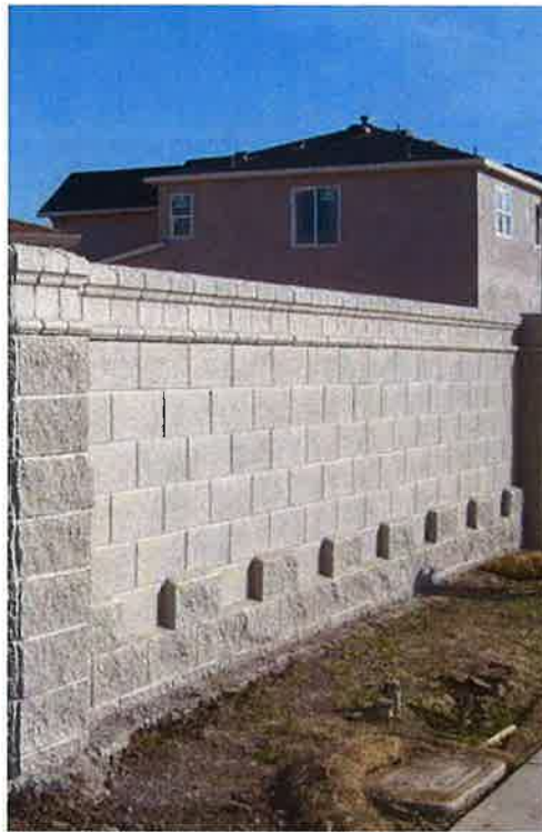
(Example of masonry block sound wall)
