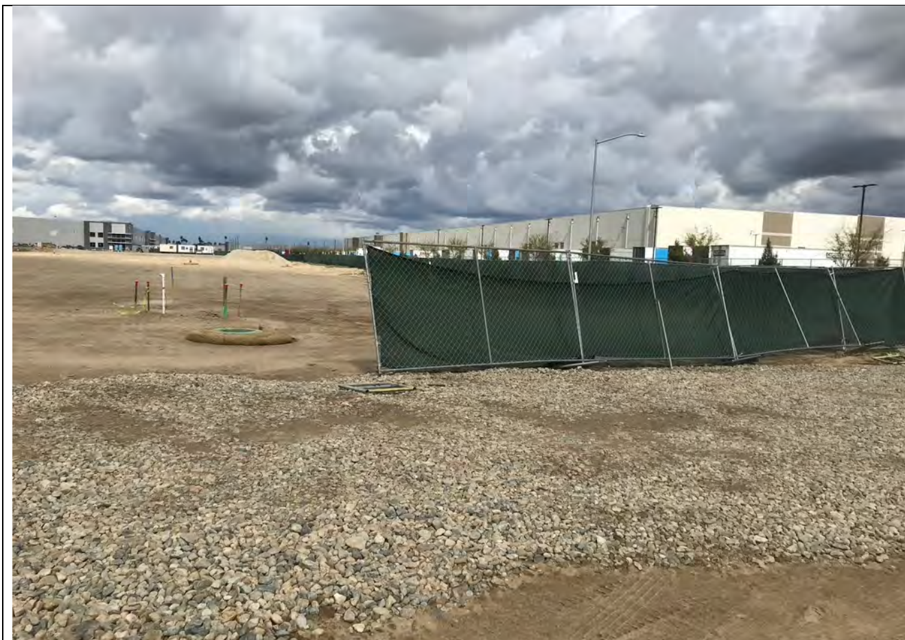
Photo 5: View of northern edge of Study Area. Gravel area is part of construction entrance.
