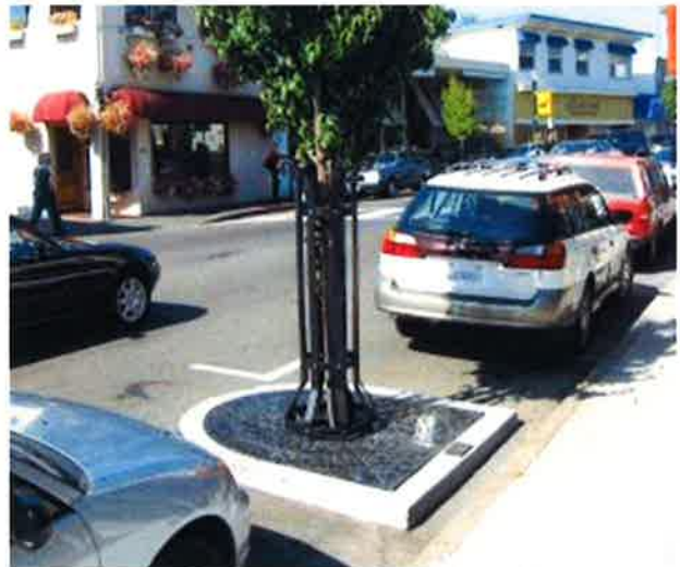
In-street tree planters can provide shade and beauty while maximizing the pedestrian walkway in areas with space constraints.
