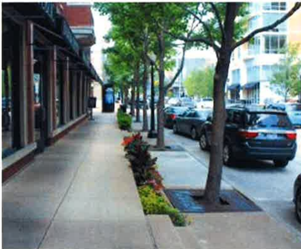
A raised sidewalk can allow for proper urban retail frontage, while still mitigating flood risk.
