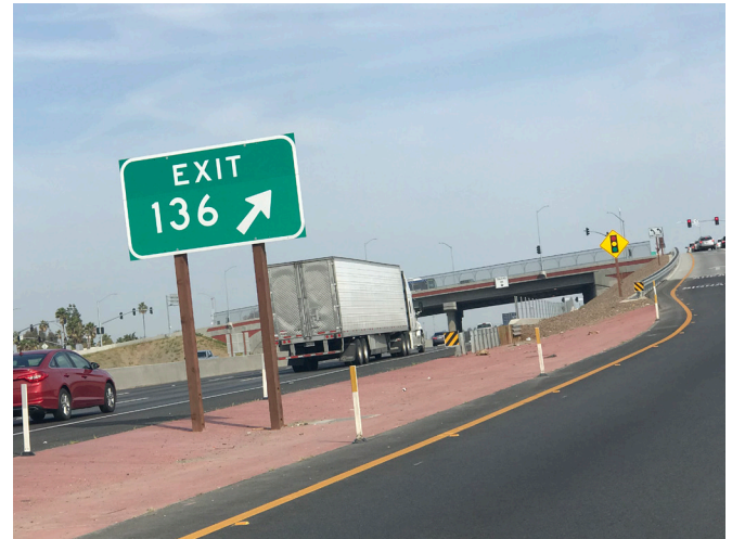
Off ramp to Clinton Ave from Highway 99.
