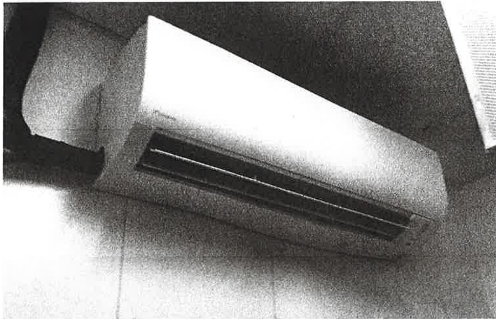
Figure 26 Mini-Split Indoor Unit
