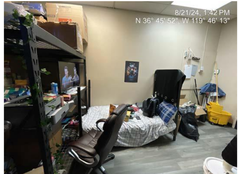
Illegal addition of habitable space
