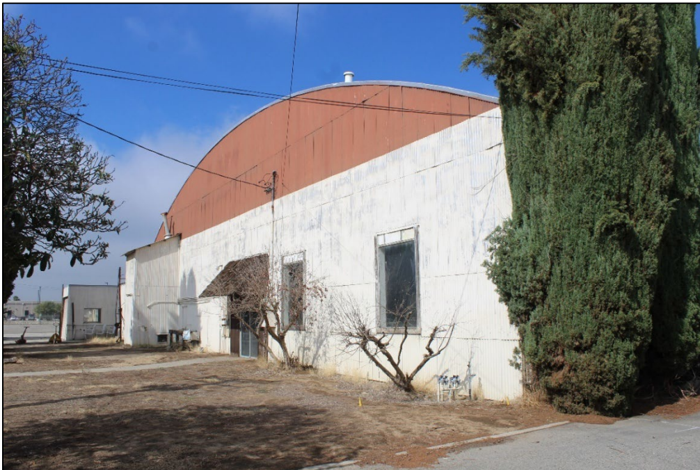
Figure 10. South façade of the hangar, facing northwest (Stantec, 2025).
