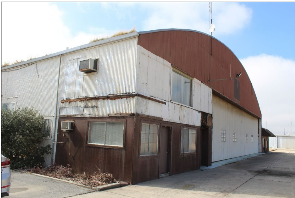
Figure 2. Northeast corner of the hangar, facing southwest (Stantec, 2025).
