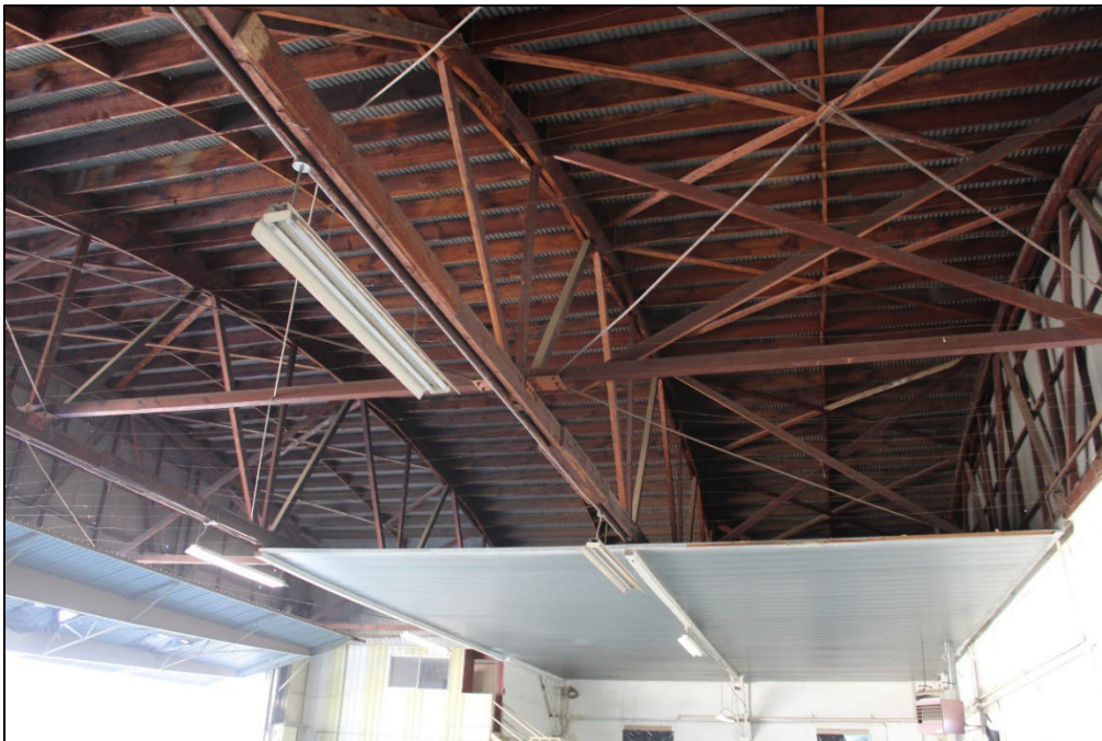
Figure 14. Wood truss frame roof inside the hangar (Stantec, 2025).
