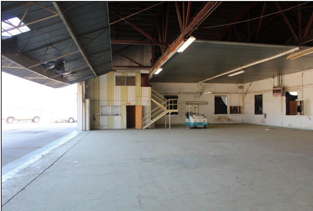
Figure 13. Interior of the hangar with hangar door open, facing east (Stantec, 2025).
