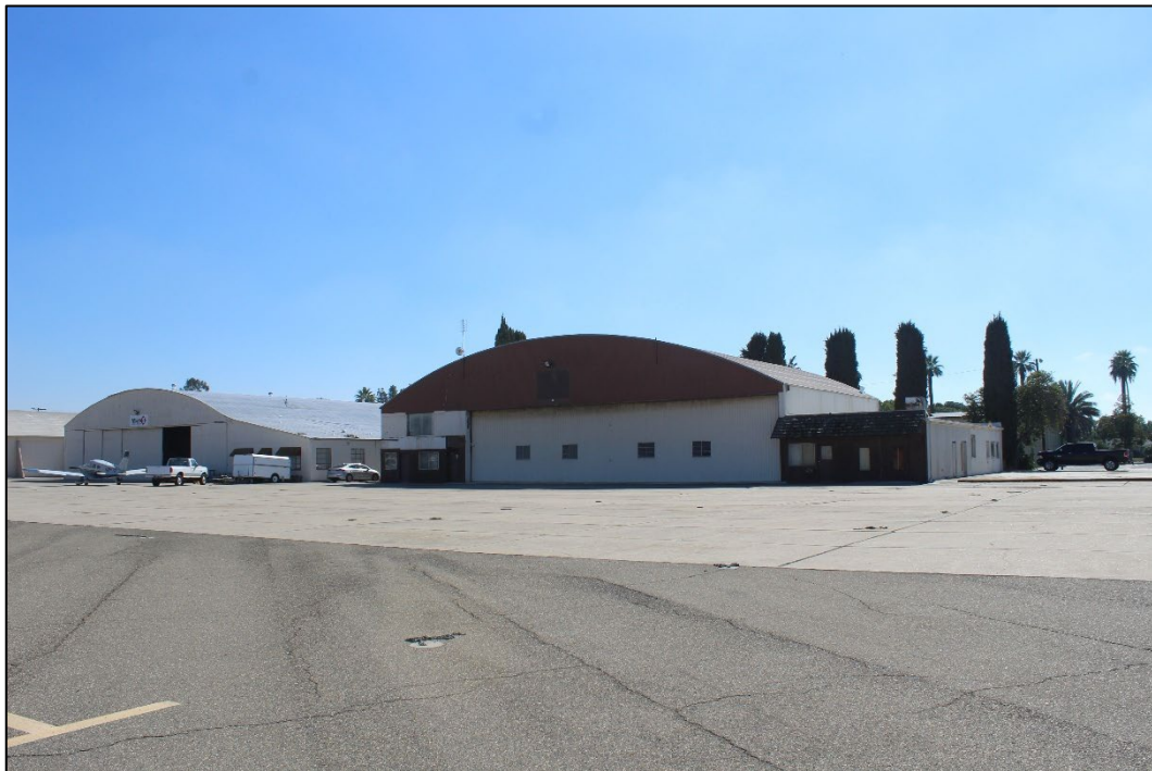
Figure 2. Hangar at 716 W. Kearney Boulevard within the Fresno Chandler Executive Airport, facing southeast (Stantec, 2025).
