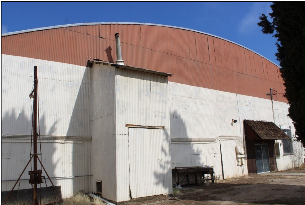
Figure 8. South façade of the hangar, facing northeast (Stantec, 2025).
