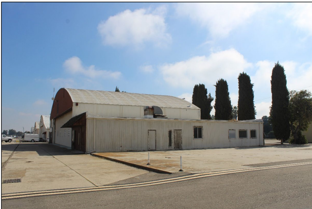
Figure 8. West façade of the hangar, facing east (Stantec, 2025).
