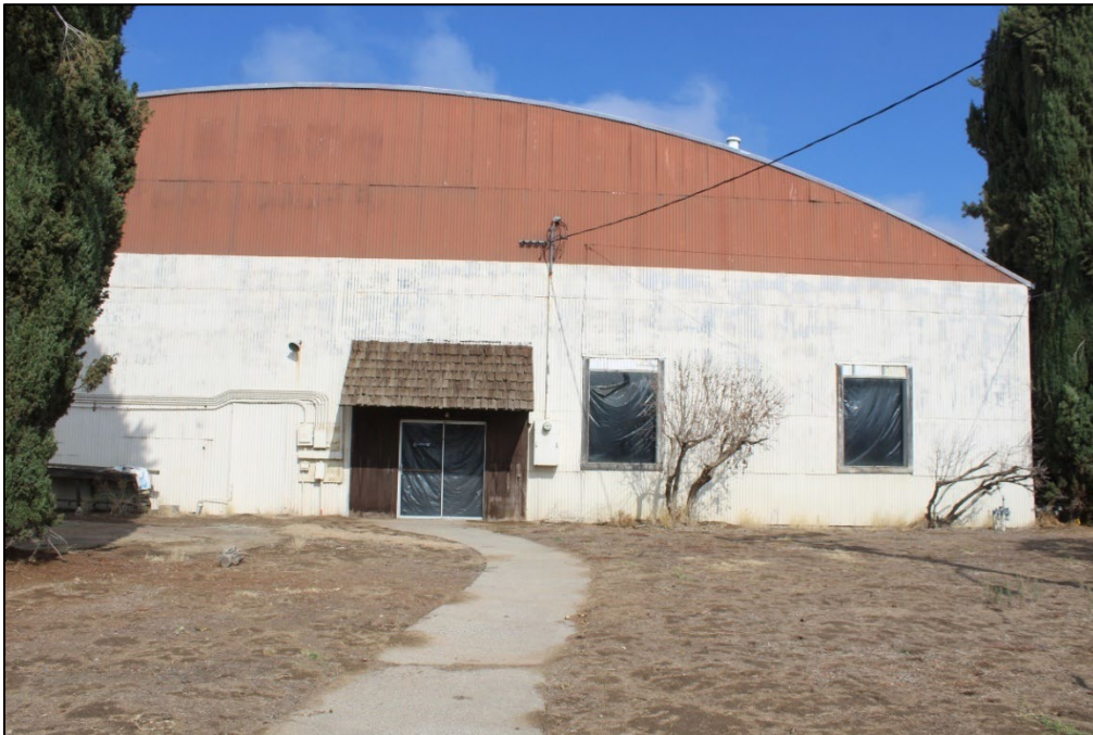
Figure 9. Entrance on south façade of the hangar, facing north (Stantec, 2025).
