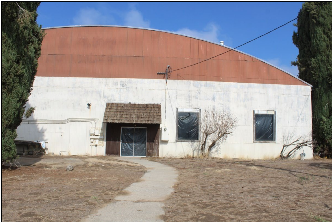
Figure 11. Entrance on south façade of the hangar, facing north (Stantec, 2025).
