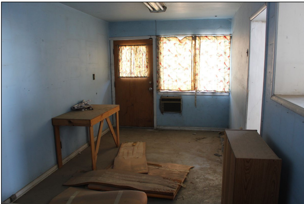
Figure 22. Interior of the addition, facing north (Stantec, 2025).
