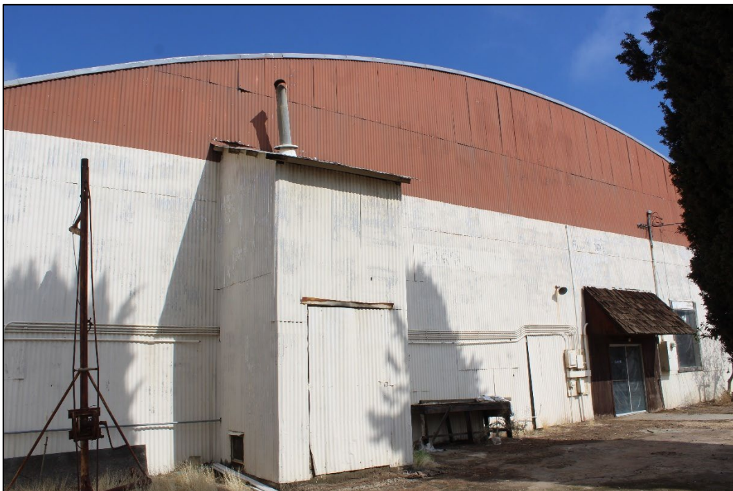
Figure 10. South façade of the hangar, facing northeast (Stantec, 2025).
