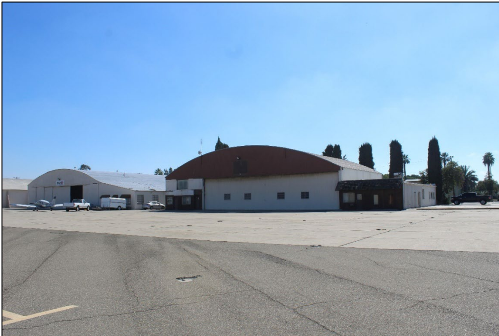
Figure 1. Hangar at 716 W. Kearney Boulevard within the Fresno Chandler Executive Airport, facing southeast (Stantec, 2025).
