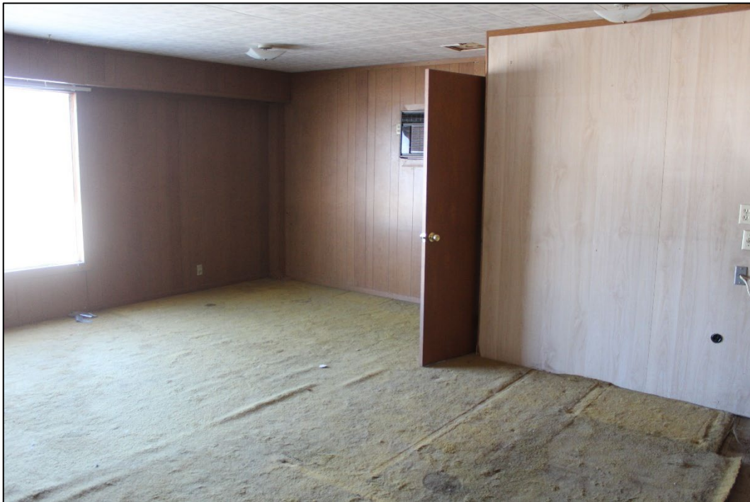
Figure 21. Interior of the apartment above the integrated office, facing northeast (Stantec, 2025).
