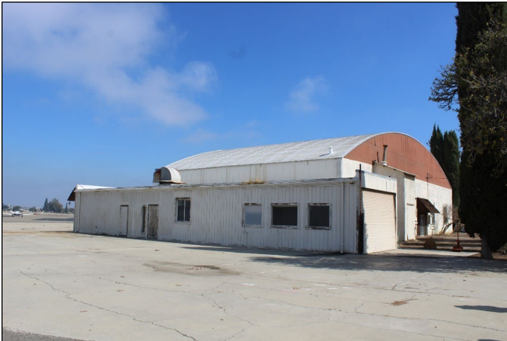
Figure 7. West and south façades of the hangar, facing northeast (Stantec, 2025).
