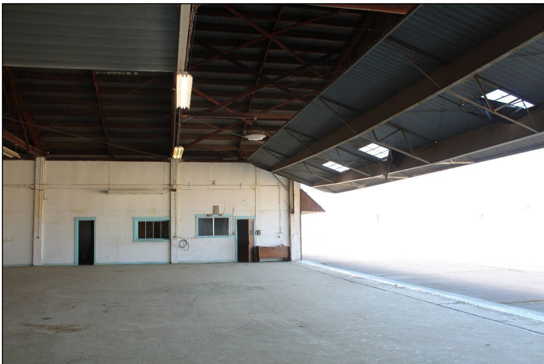
Figure 14. Interior of the hangar with hangar door open, facing west (Stantec, 2025).
