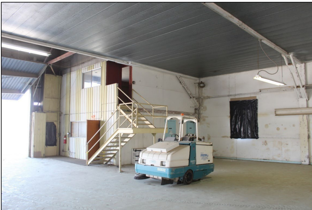
Figure 16. View of the integrated office and apartment from inside of the hangar, facing northeast (Stantec, 2025).
