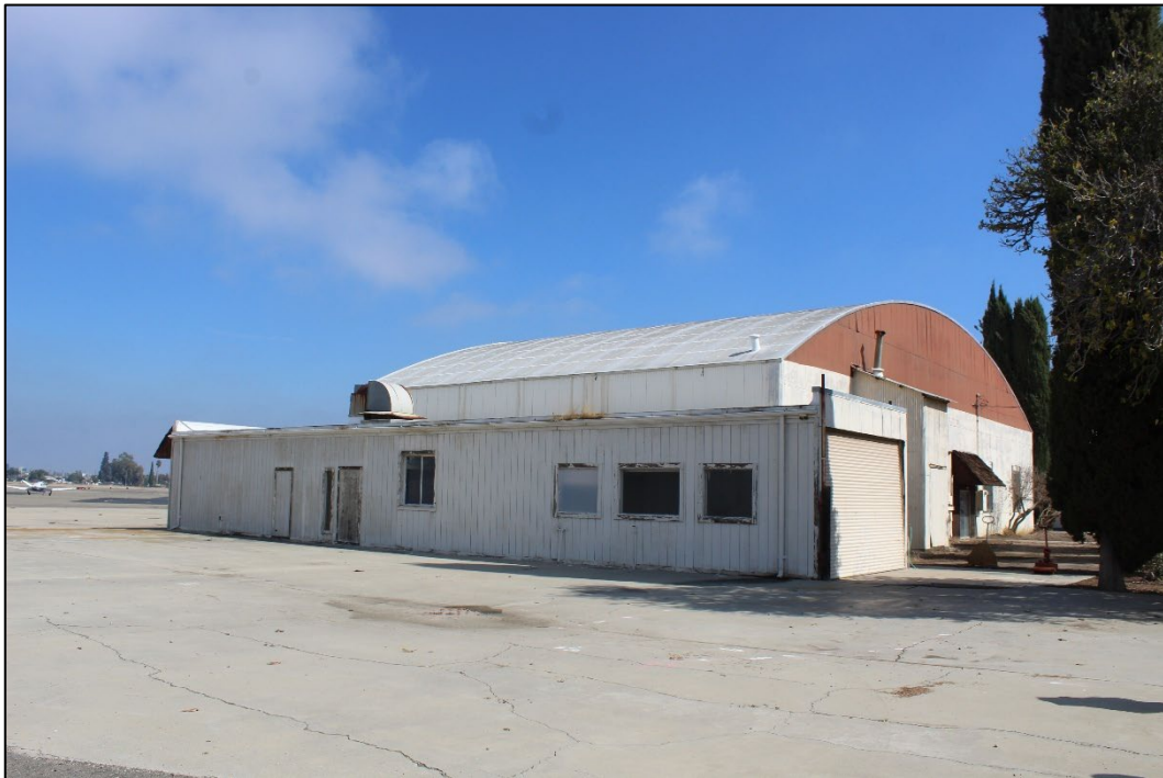
Figure 9. West and south façades of the hangar, facing northeast (Stantec, 2025).
