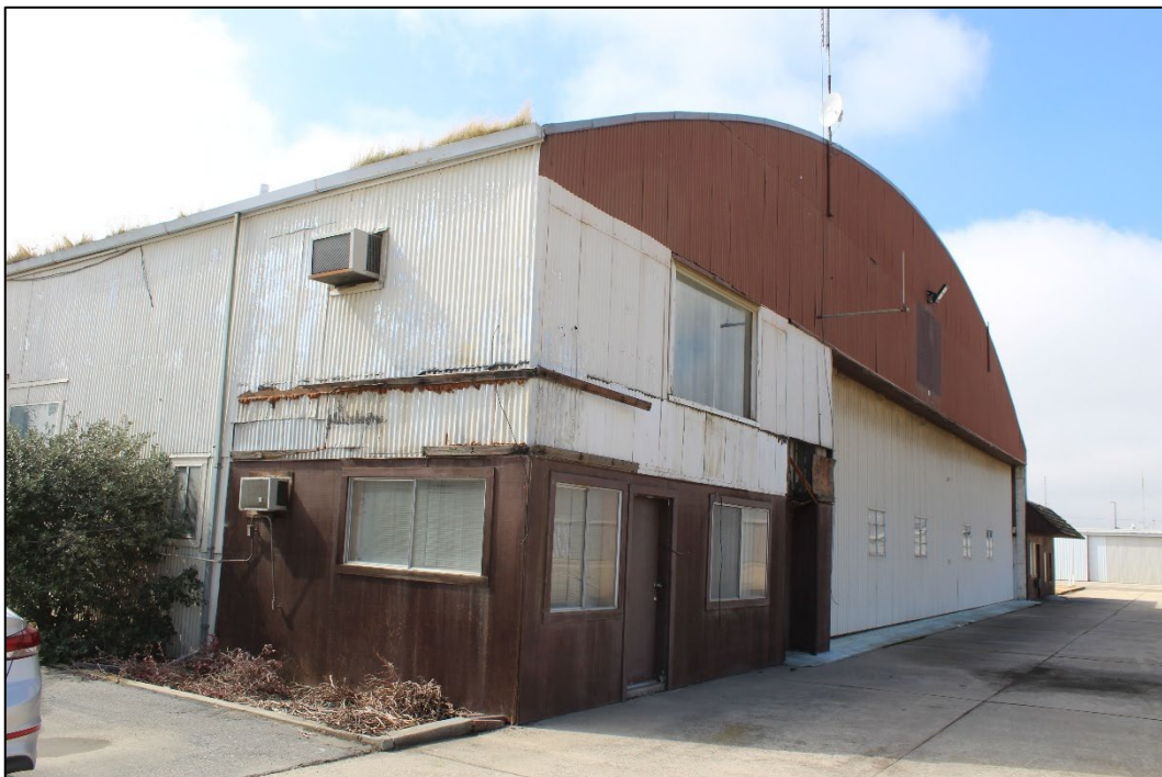
Figure 4. Northeast corner of the hangar, facing southwest (Stantec, 2025).
