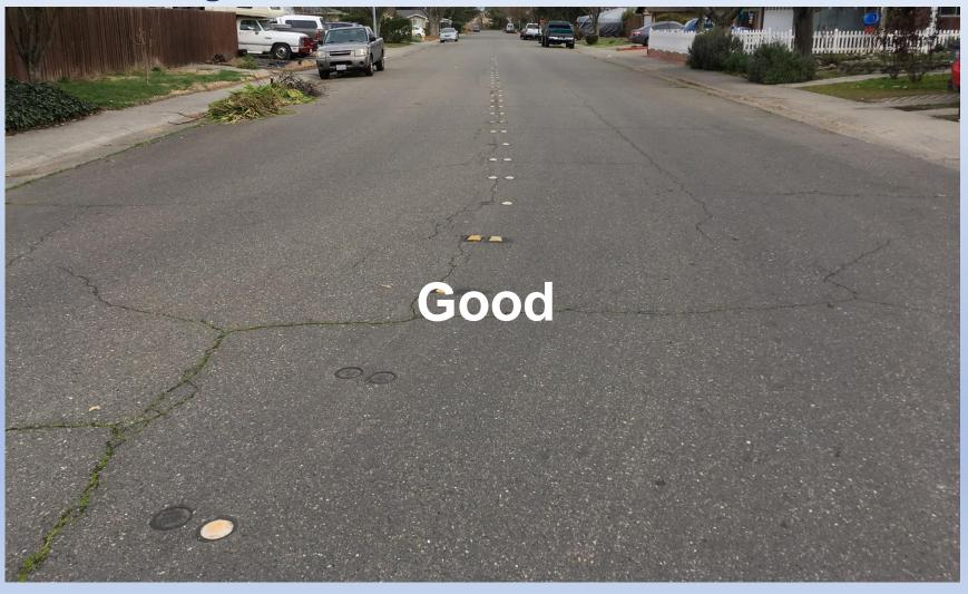
**Network** PCI = 75**Treatment is** crack and slurry seal
