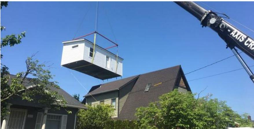
***An example of a prefabricated ADU<sup>1</sup> being craned into a residents backyard.***
