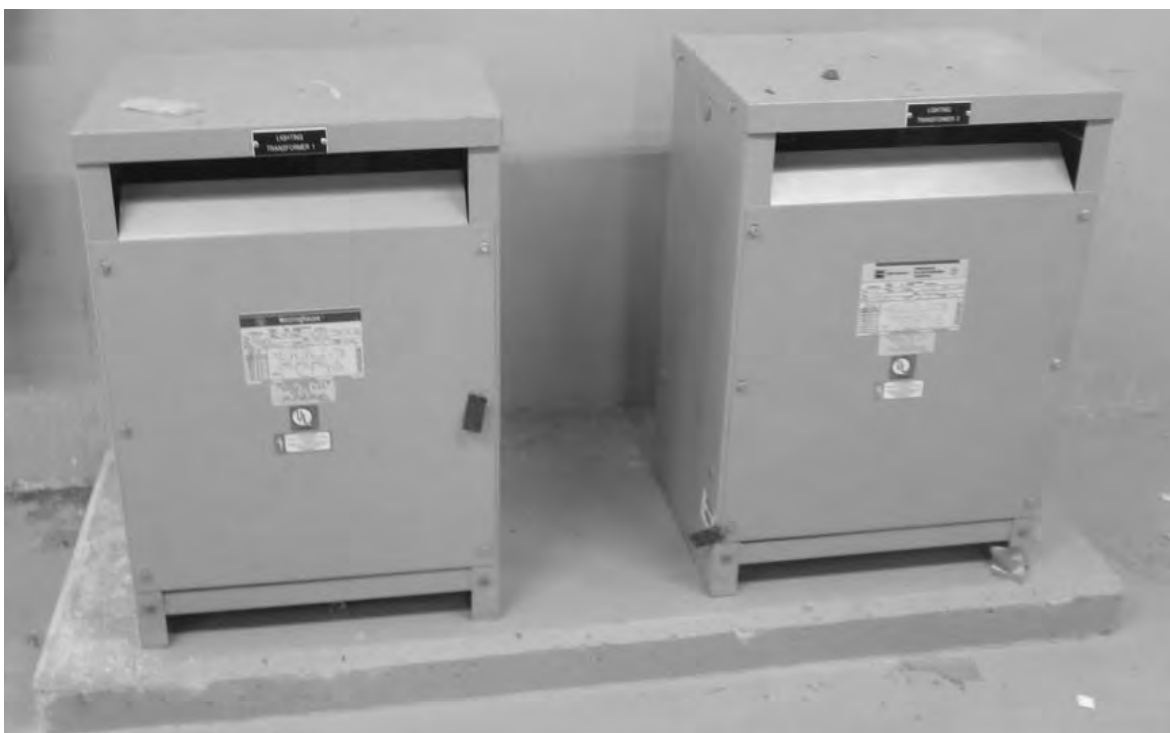
Headworks: Lighting Transformer T-1 and T-2
