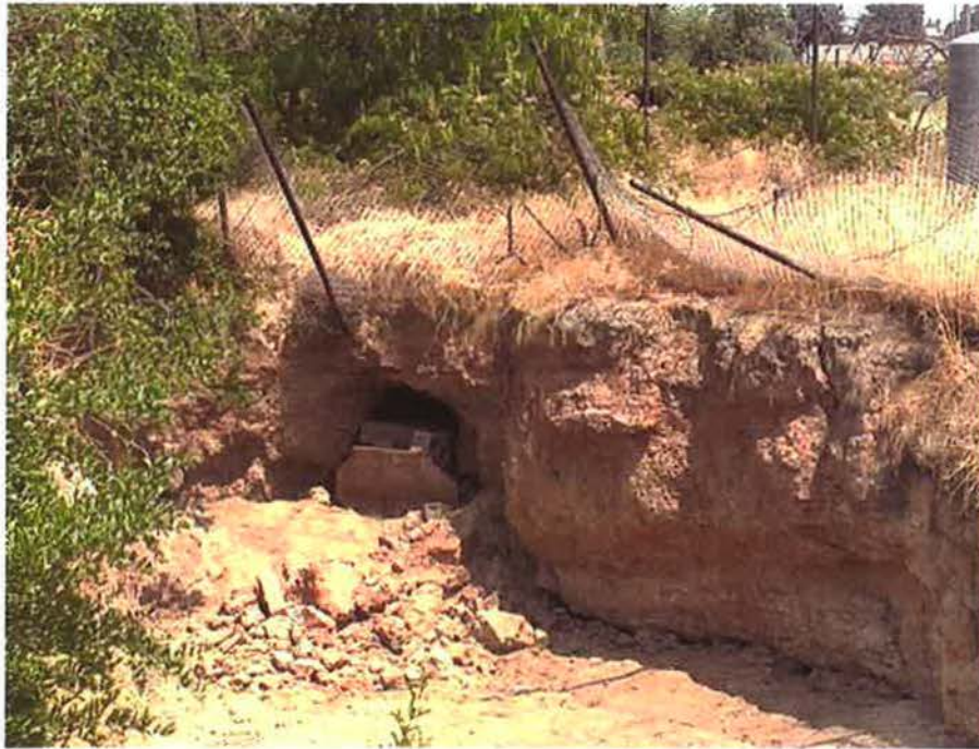
Figure 6: Photo (facing east) of excavated "stair tunnel" entering the eastern 10 acre parcel from an excavated area in the Forestiere Underground Gardens. The tunnel was not entered during this project, but GPR transects crossed it on the grassy area between the fence and trees. This is Area of Interest A.
