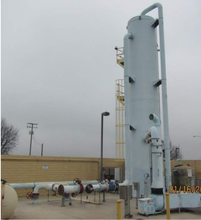
Photo 8: Packed Tower Aerator
