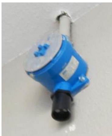
Photo 2: Gas Monitoring Device in Site Office
