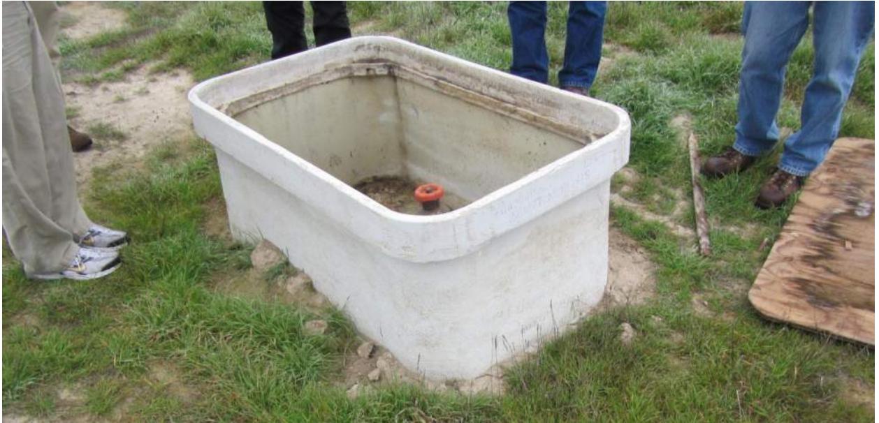
Photo 22: Gas Extraction Wellhead. Note the subsidence, as rim of well box was once at grade.
