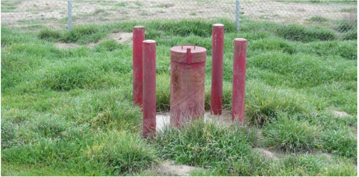
Photo 20: Perimeter Gas Well
