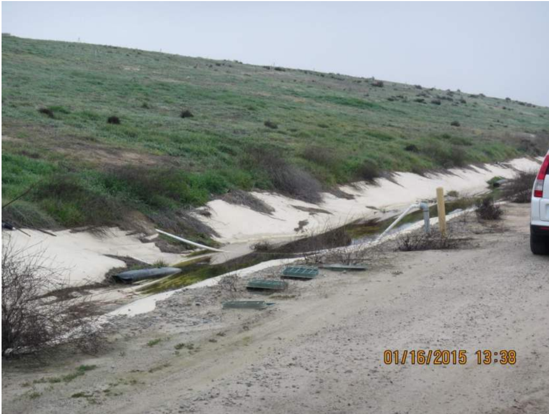
Photo 26. Surface drainage ditch on the east side of the landfill. Due to subsidence, ditch is now lined.
