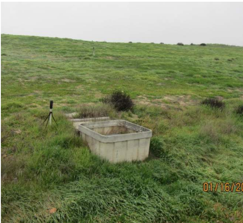
Photo 11: Landfill Gas Condensate Sump
