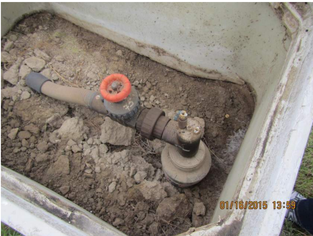
Photo 21: Gas Extraction Wellhead
