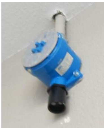
Photo 2: Gas Monitoring Device in Site Office
