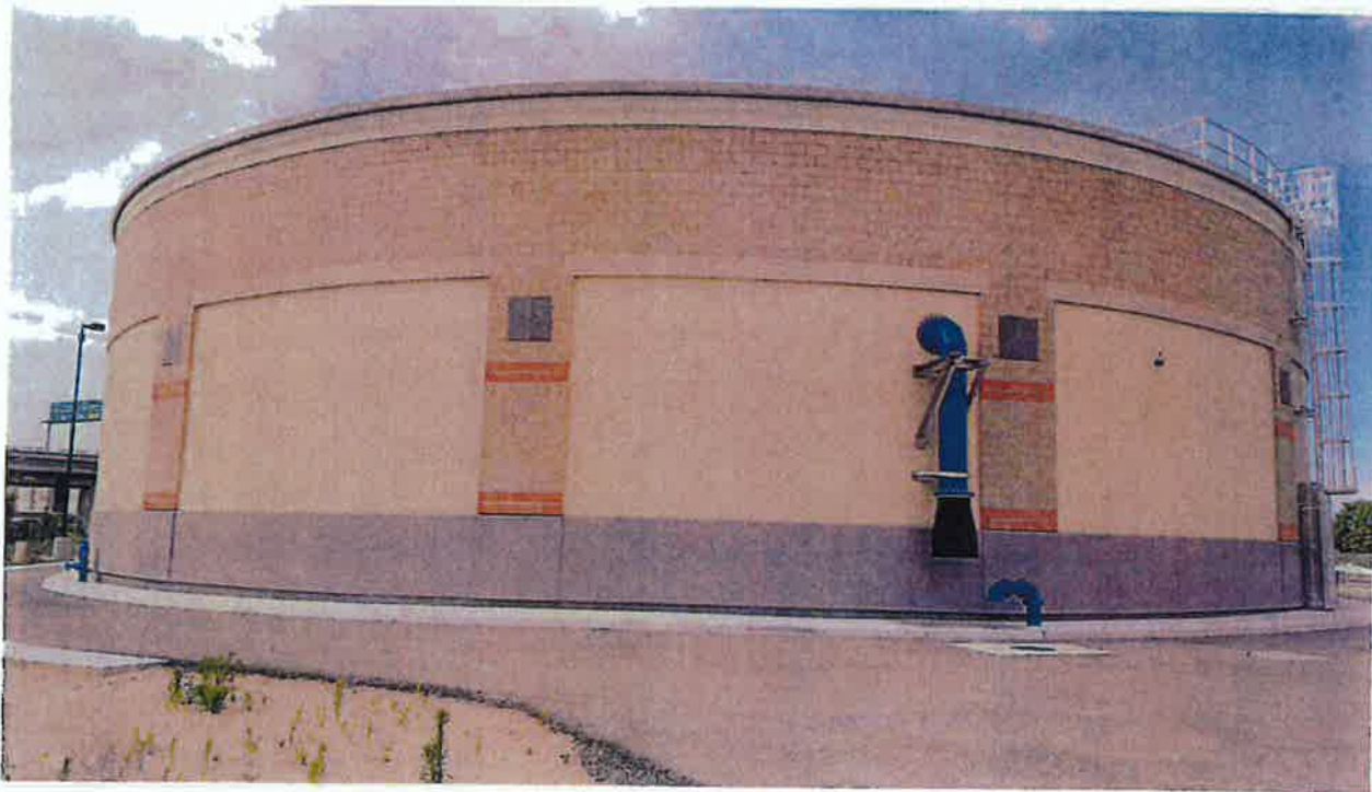
Completed T-4 3 MGD Tank by Mountain Cascade, Inc. for the City of Fresno
