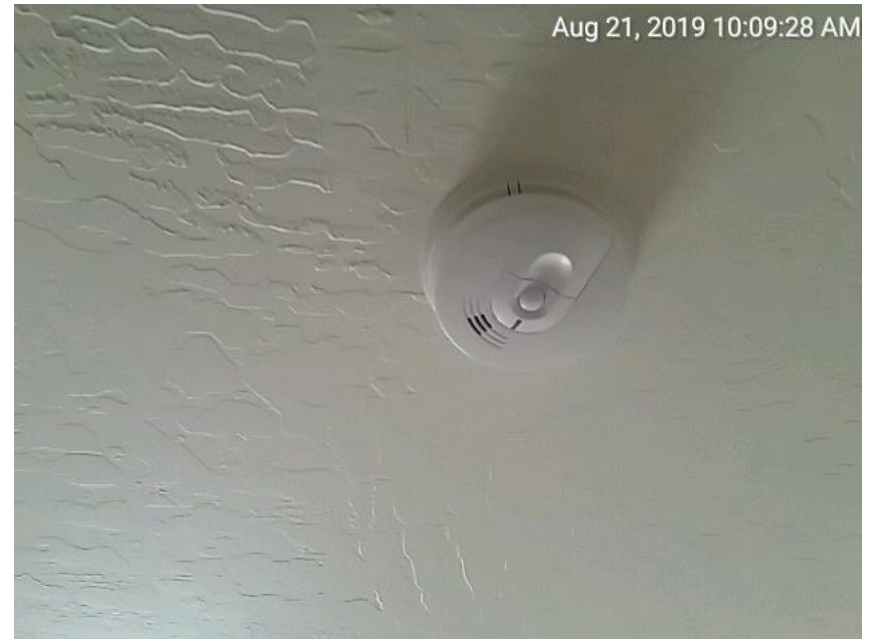
Smoke detector install in bedroom
