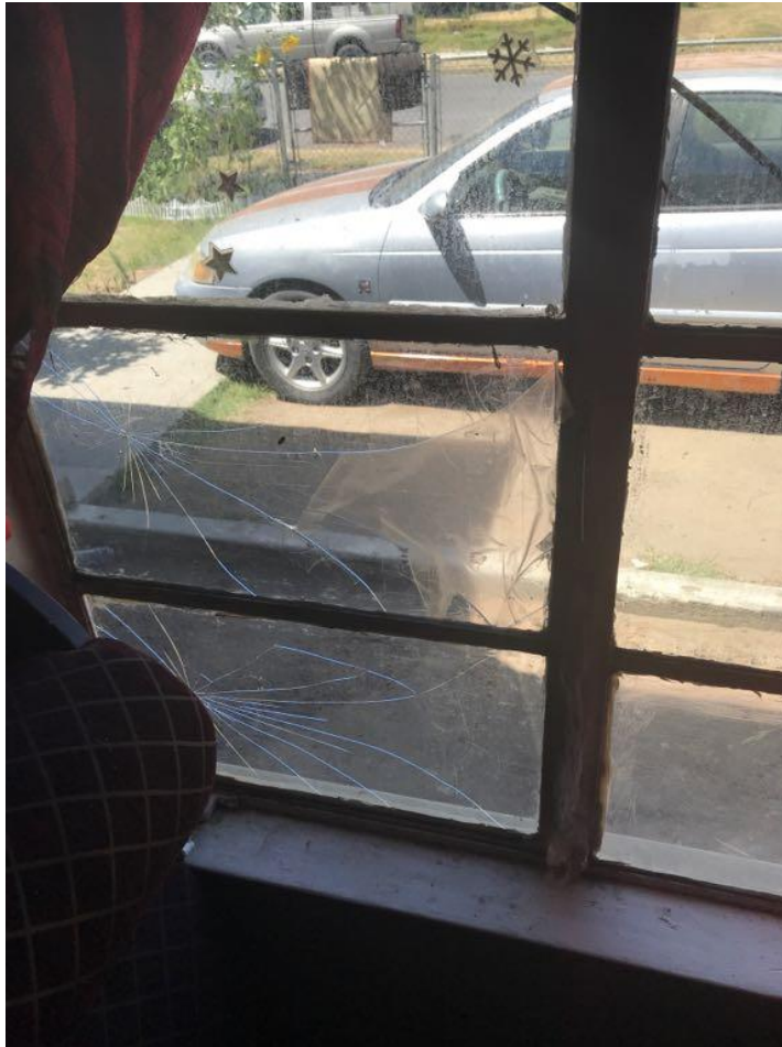
Living room – Windows / Window Locks (Windows intended for opening can be opened and locked, no missing or broken glazing, egress not blocked, security bars can be released from the interior). Window Broken
