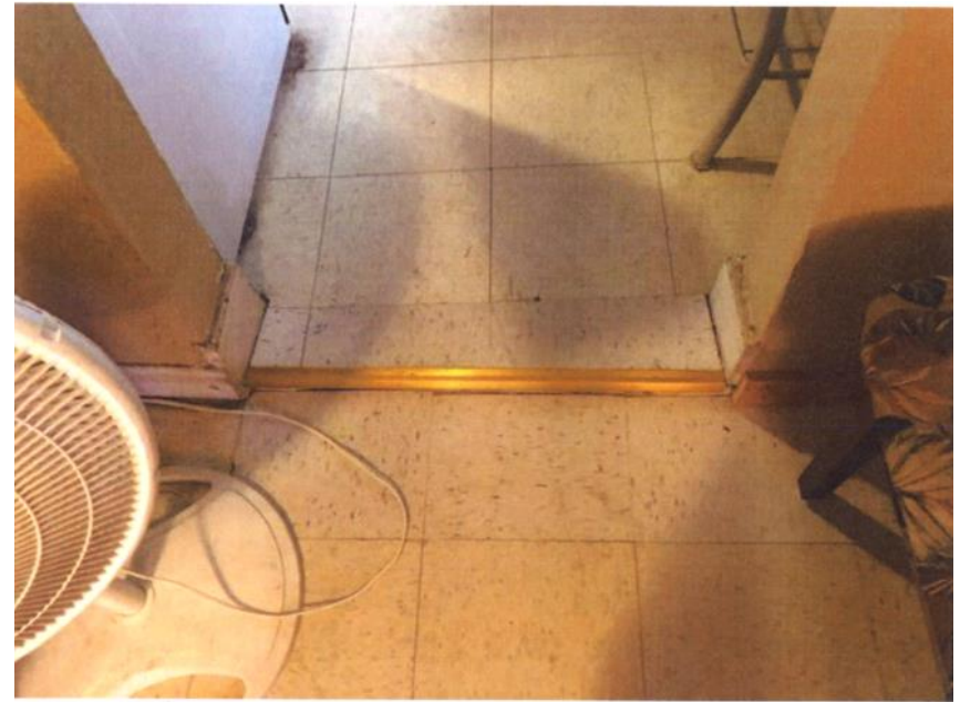
Broken floor tiles replaced and threshold installed.
