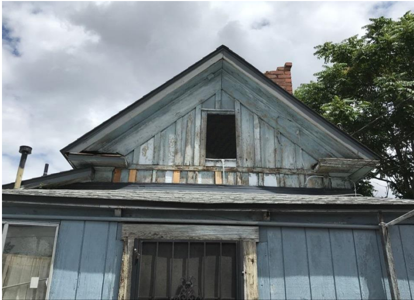
Exterior – Exterior Walls without Effective Waterproofing and Weather Protection. Lack of waterproofing and weather protection posing health concerns.
