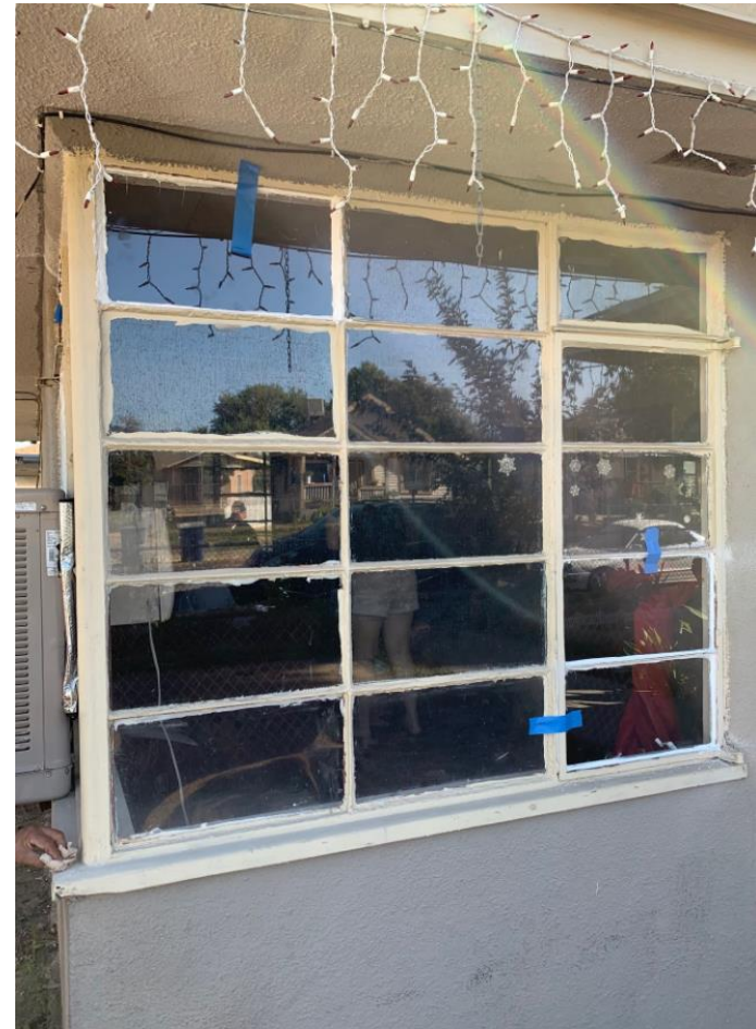
Broken pane windows replaced.
