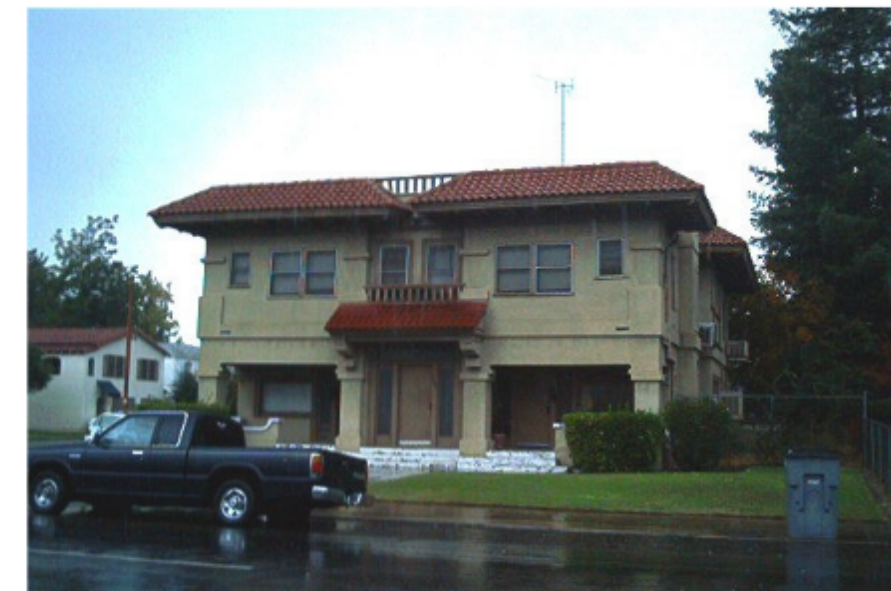
Tower 4-Plex at Wishon and McKinley.
