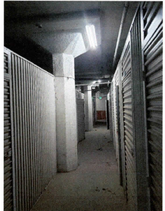
Interior of building near office.
