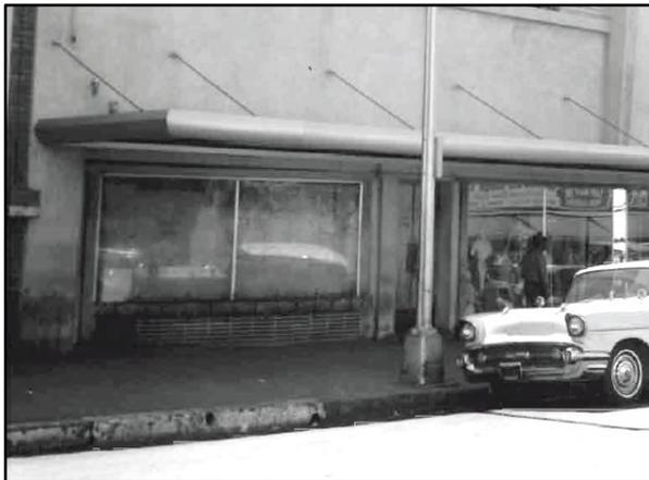
**Figure 52. The storefront window and brick bulkhead at the southeast end of the building are shown above in 1966 (Fresno Public Library).**
