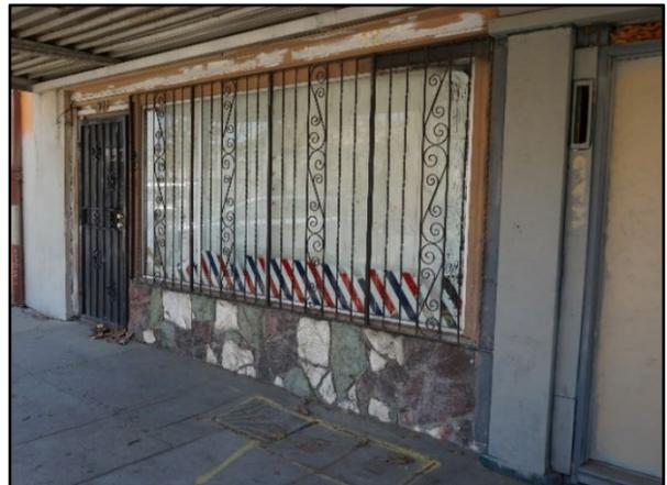
**Figure 53. A 2024 photograph above shows the added door (left) and stone veneer (SWCA 2024).**
