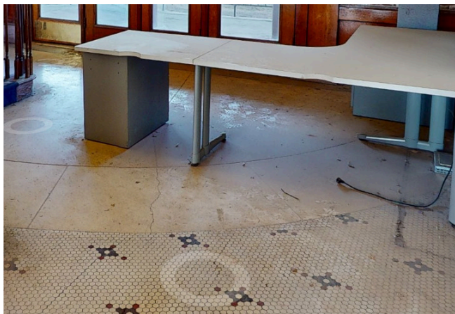
Existing Terrazzo floor (semicircle shape) at south doors
