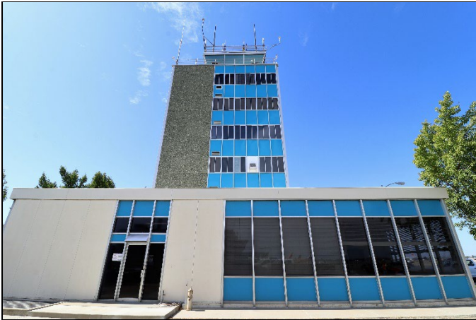
Southeast (side) elevation, view northwest (9/11/23).
