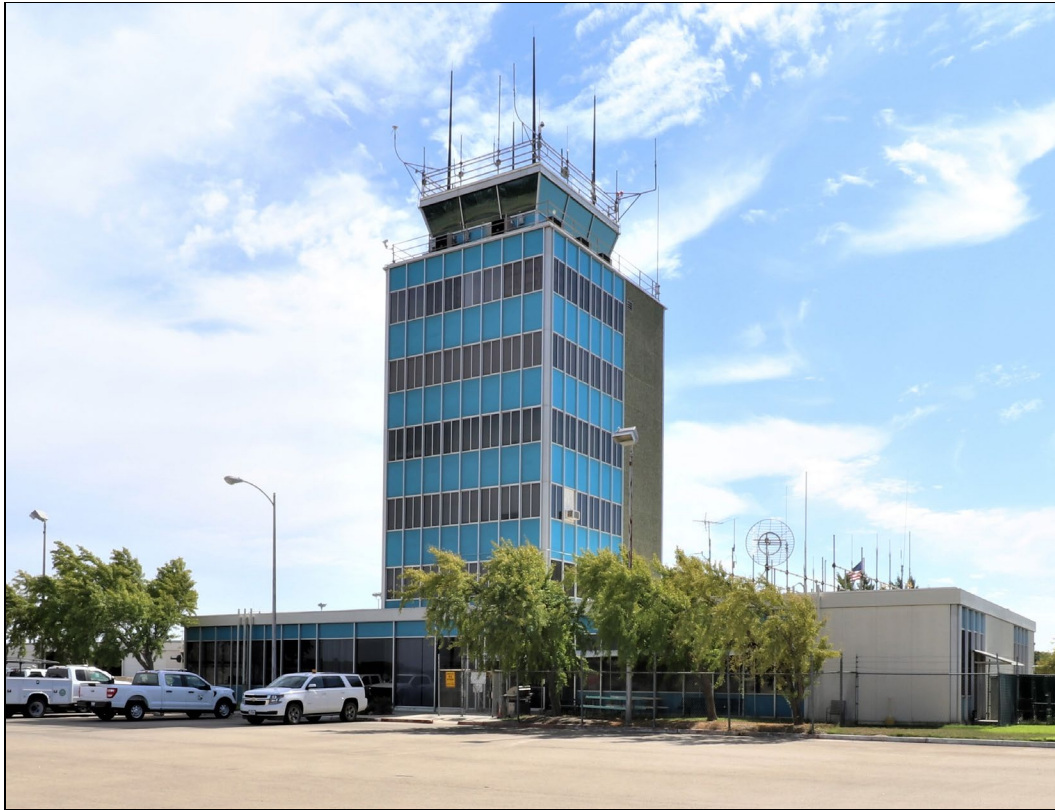
Photo 4: Northeast elevation, view south (9/11/23).
