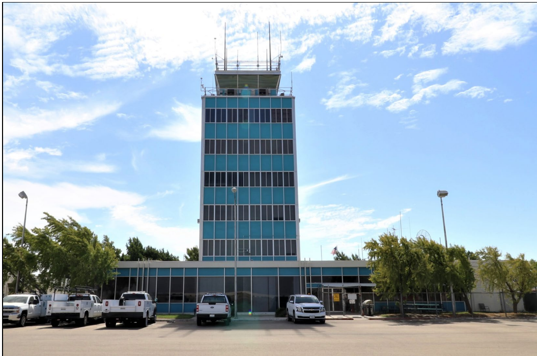
Photo 3: Northeast elevation, view southwest (9/11/23).
