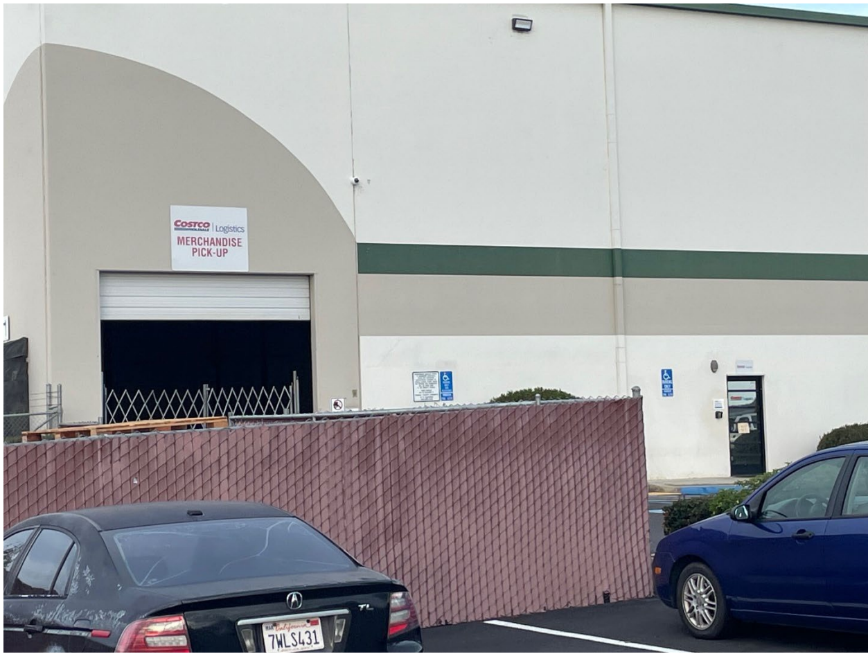
Image of entryway area of existing Costco Logistics Merchandise Pick-Up Facility
