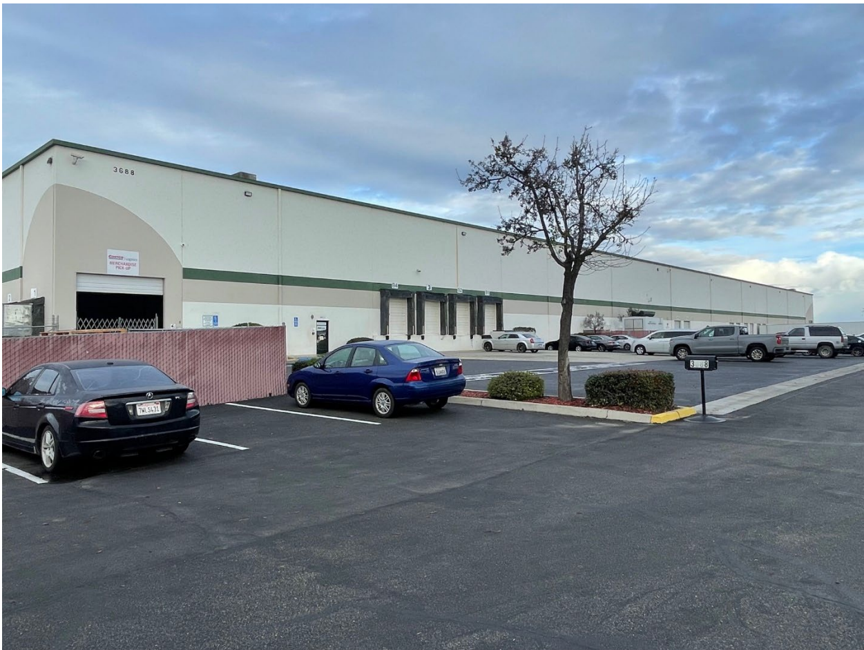
Image of existing Costco Logistics Merchandise Pick-Up Facility (front/south side)
