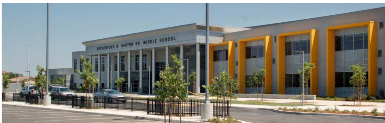
Recently constructed Gaston Middle School.
