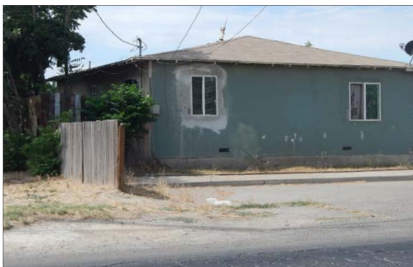
Inconsistent sidewalks in a Southwest Fresno neighborhood.
