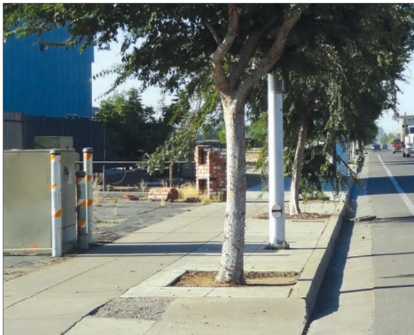
Existing sidewalk with street trees.
