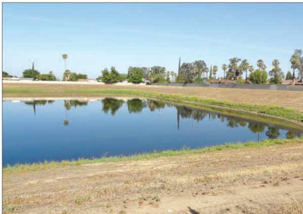
Ponding basins collect water to manage stormwater runoff.
