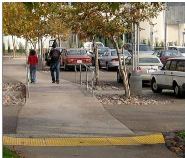
Pedestrian pathways through parking areas help people feel safer walking to destinations.
