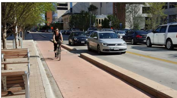
Class IV cycle track with a physical barrier providing separation from traffic.
