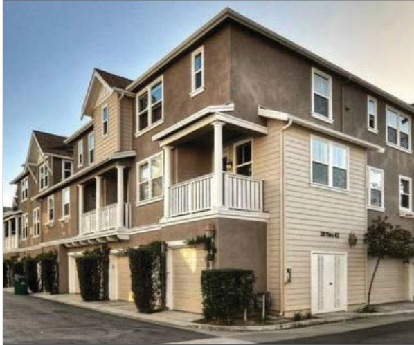
Urban Neighborhood residential creates compact development with multi-family dwellings.
