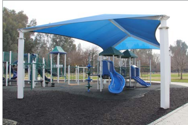
Playground with overhead shade structure.
