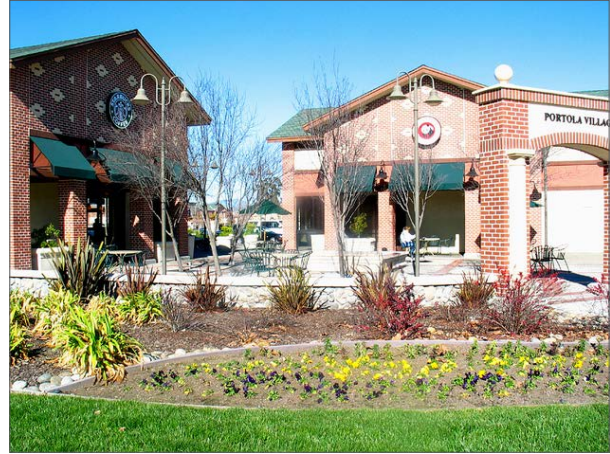
Shopping center with entryway, pedestrian plaza, lighting, attractive materials, and signage.
