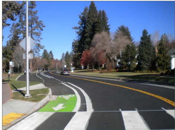
Street with Class II bicycle facilities and a high-visibility crosswalk.
