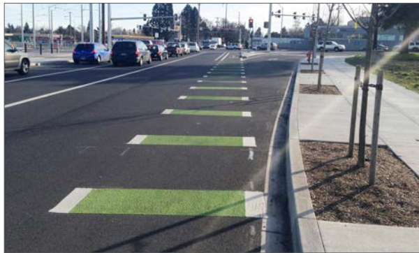
Broken Class II green bike lane to allow vehicles to cross through.
