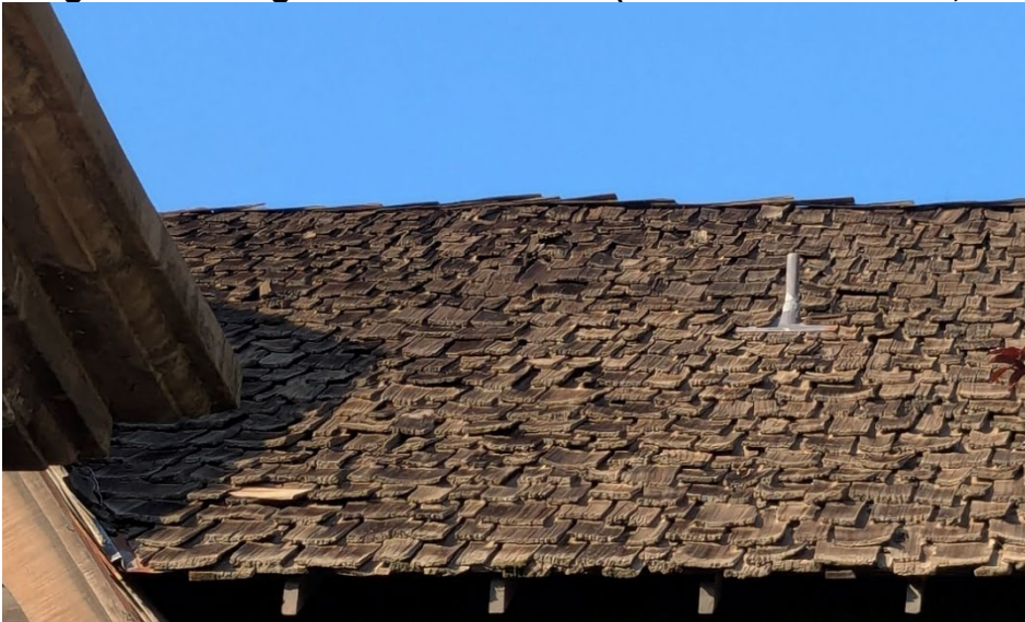
Image 2: Existing Wood Shake Roof (Source: Staff Photo, October 2024)
