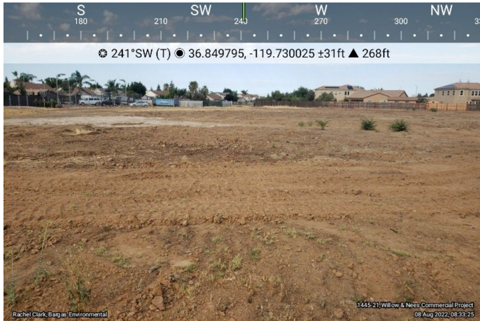
Photo 5. Graded pad where structure was removed from. Also visible is open ground which may be attractive to certain ground nesting birds.
