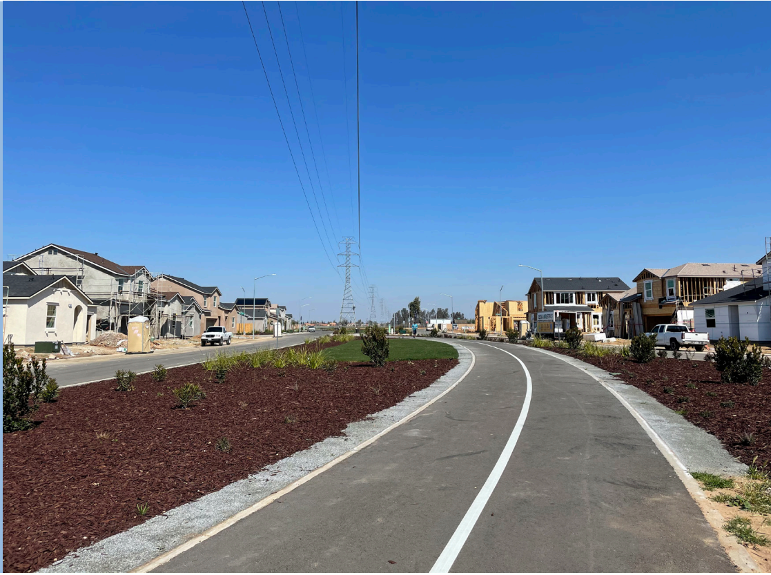
A Class I Bike/Pedestrian Path along Gorma Avenue is a prominent feature of this future neighborhood
