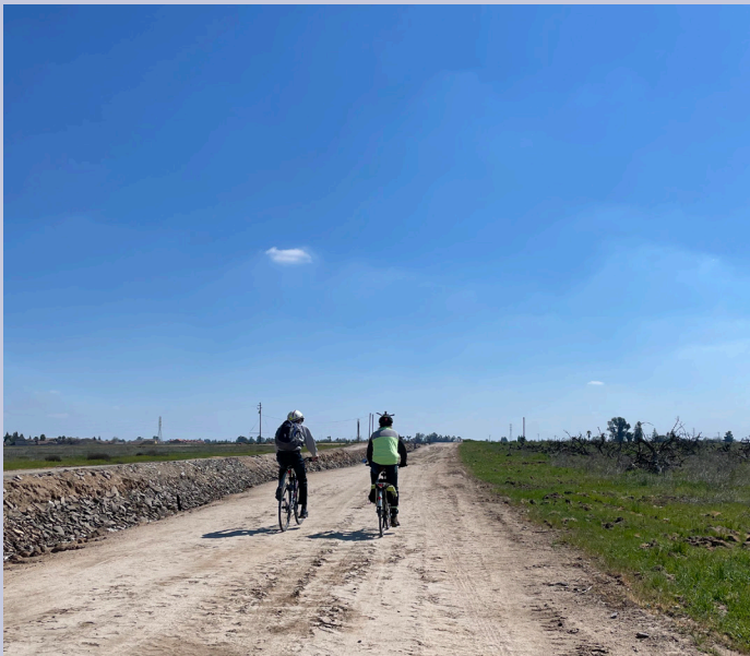
Herndon Canal in the West Area
