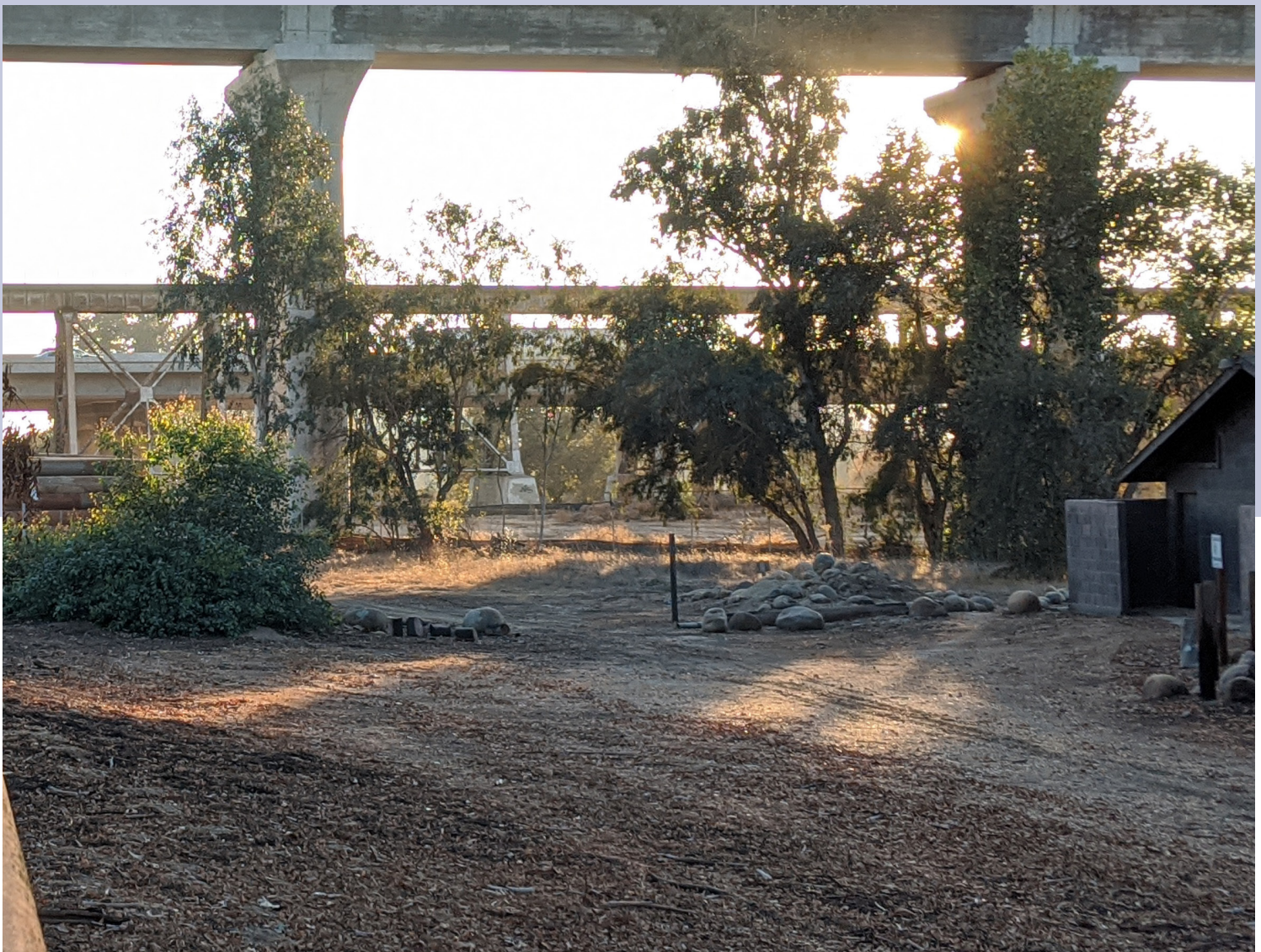
View looking west under Highway 99 and train bridges by the San Joaquin River
