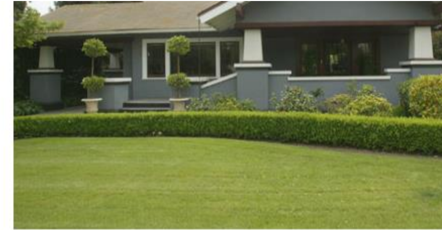
Hidden Equipment. This residence's HVAC unit is not visible from the street.
