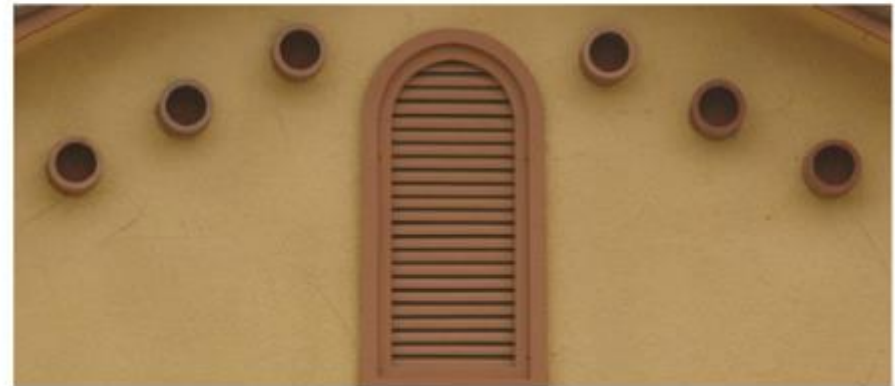
Attic Vents. Common attic vent types in the Tower District.
