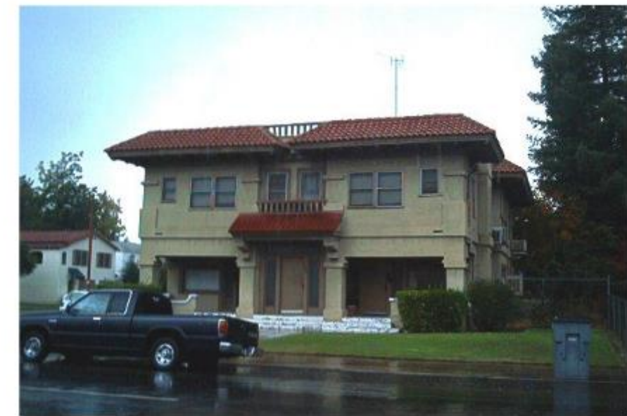
Tower 4-Plex at Wishon and McKinley.
