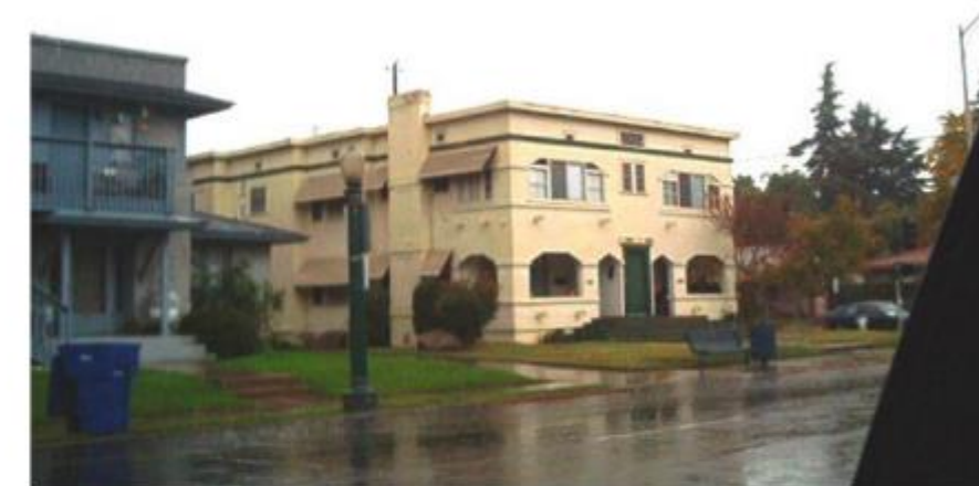
The parking lot for this apartment house is behind the main structure, accessed by a driveway along the side of the building. This is the preferred placement for Multiple family parking.
