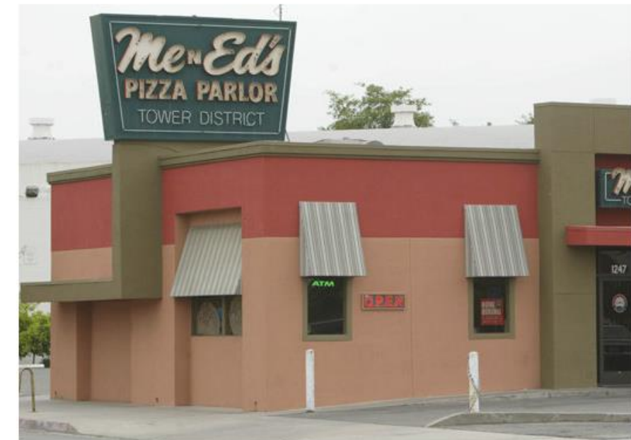
Roof Signs. This roof sign exemplifies the architecture of this building.
