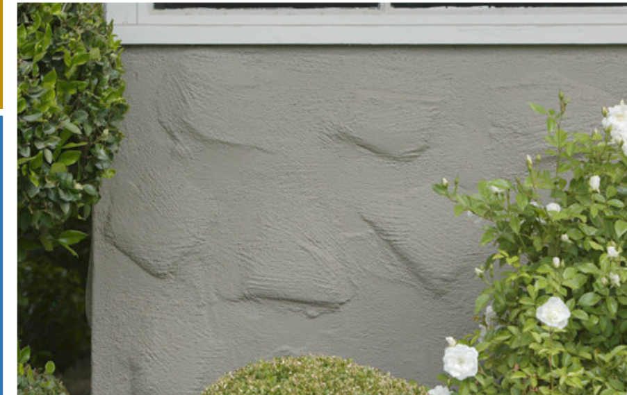
Appropriate Stucco. This unique stucco application is appropriate for this early ranch house. However, it would be inappropriate on a Craftsman style home.
