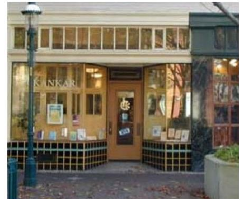
Recessed Storefront Entrance. Doors into retail spaces may be recessed within the façade, as is done in this building. Note also that the entry is located at the same exact grade as the sidewalk, which is the preferred approach.
