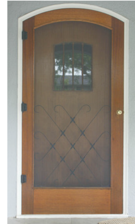
Screen Doors. Unlike a metal security door, this screen door is appropriate for this single family residence.
