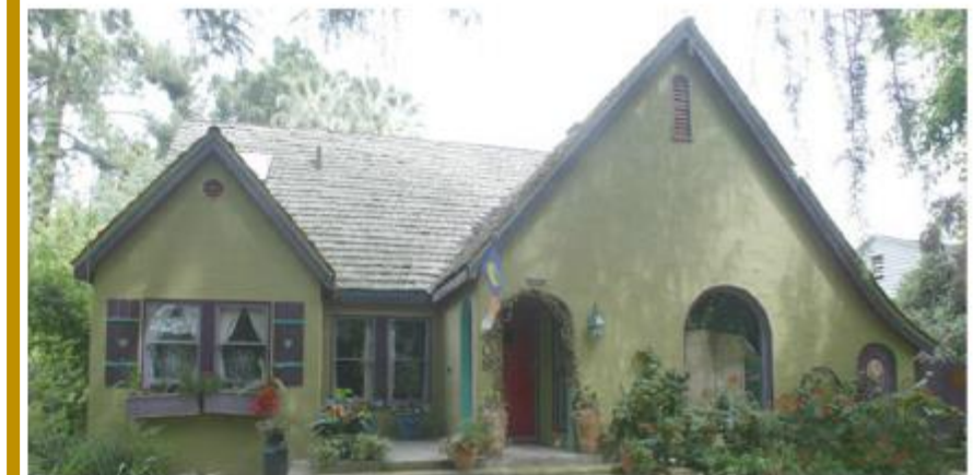
Roof Forms. The steep pitch and crossed gables of this Tudor home are key components to its architecture. Additions to this type of residence should maintain the same roofline.
