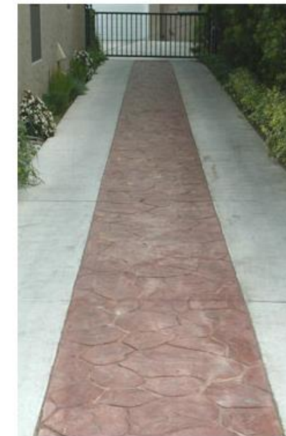
Ribbon Driveway With Alternative Materials. This photo shows good use of acceptable alternative materials for ribbon driveways.
