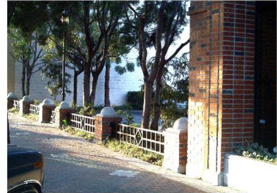
Parking Lot Screening Wall. Parking lots which are located adjacent to a street should be bordered by a screening wall.
