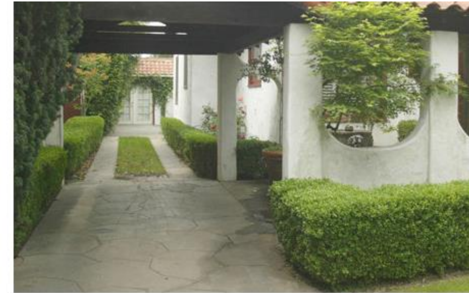
Carports. Architecturally, these carports appear to be an extension to the residence since the columns and roof materials of the main residence are consistent in the carport.
