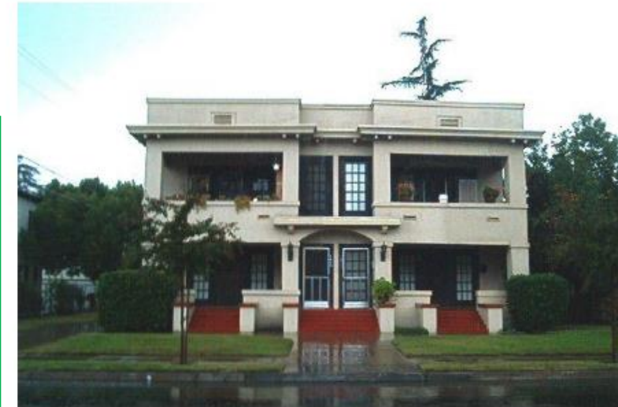
Facade Elements. This Tower District apartment house shows good use of balconies, porches, stoops, cornices, and internal stairways.
