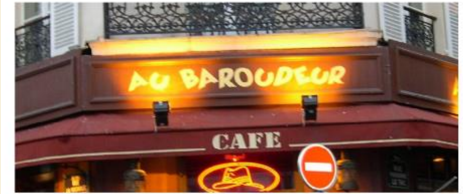
This wall sign fits completely within the frieze area and does not obscure any architectural features of the building.
