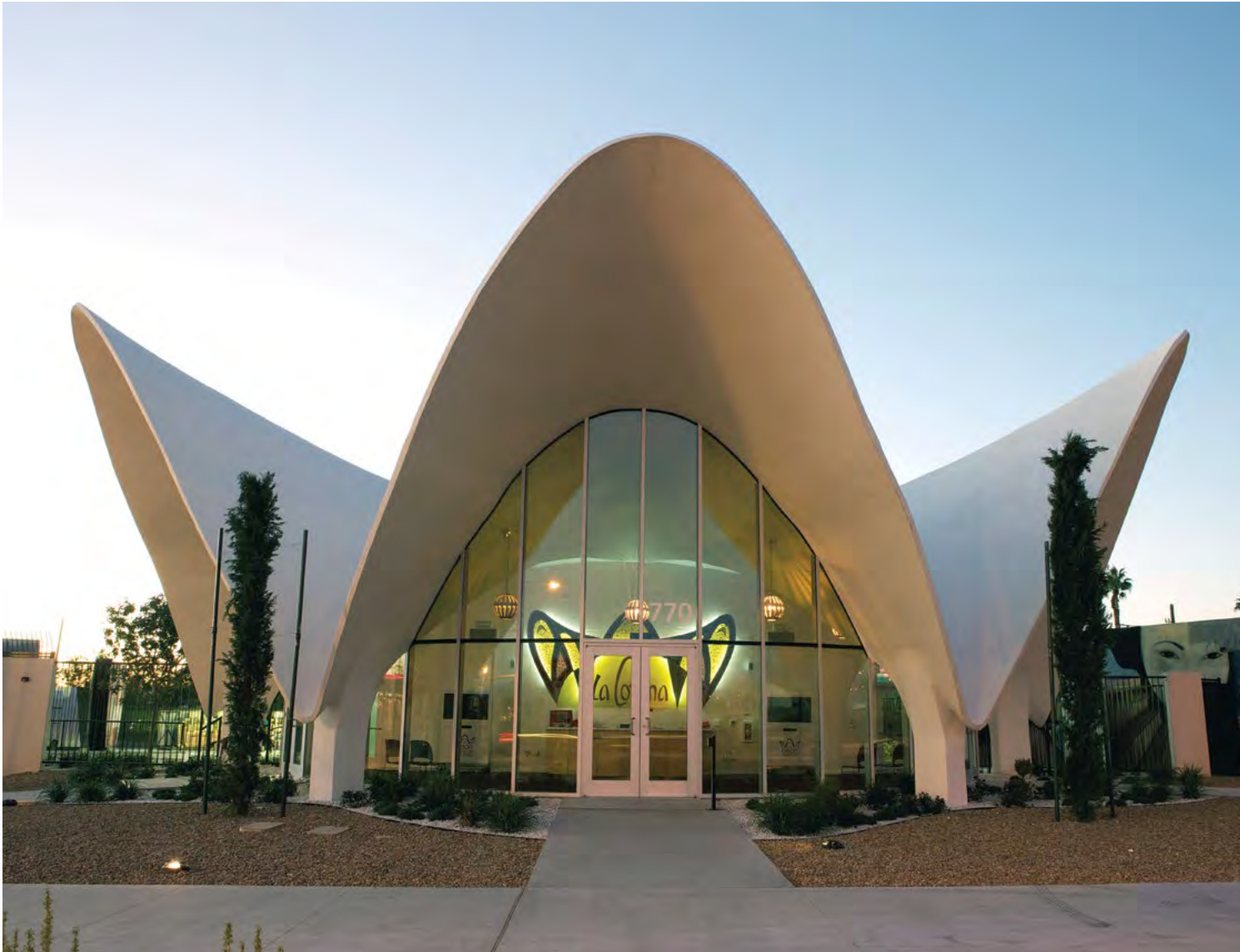
[2] Mid-century modern building technology made possible the form of this parabola-shaped structure and its thin concrete shell construction. Built in 1961 as the lobby of the La Concha Motel in Las Vegas, it was designed by Paul Revere Williams, one of the first prominent African-American architects. It was moved to a new location and rehabilitated to serve as the Neon Museum, and is often cited as an example of Google architecture. Credit: Photographed with permission at The Neon Museum, Las Vegas, Nevada.
