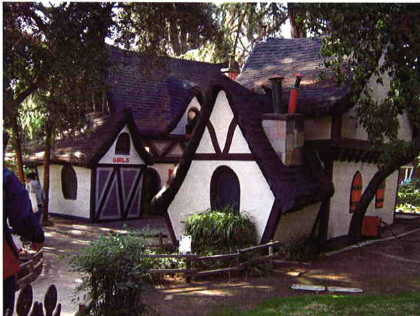
View of Restrooms (Page & Turnbull, 11/2008)
