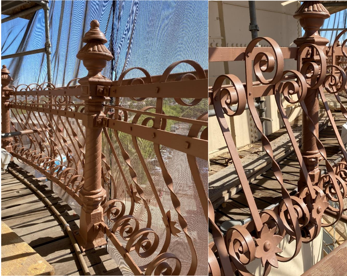
Figure 2: Existing Wrought Iron Guardrail along Upper-level Catwalks (painted Autumn Tan)
