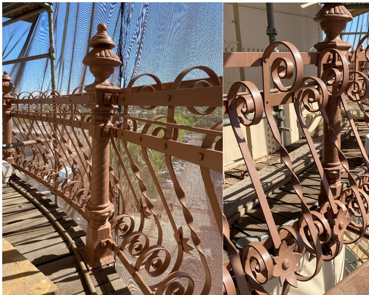
Figure 2: Existing Wrought Iron Guardrail along Upper-level Catwalks (painted Autumn Tan)
